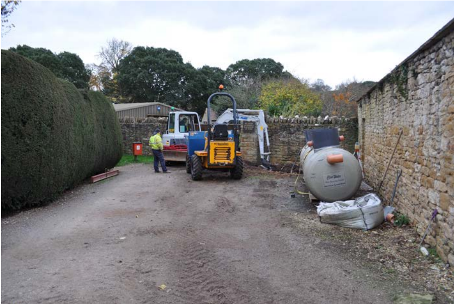
Plate 1: General View of site looking south during excavation of Trench 1.
