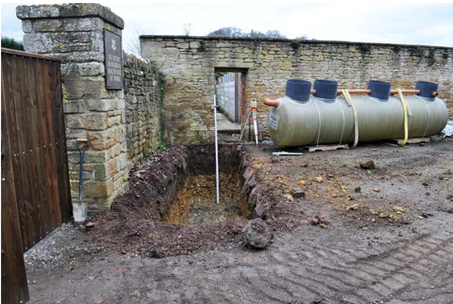
Plate 2: Trench 1 after excavation, viewed from east.
