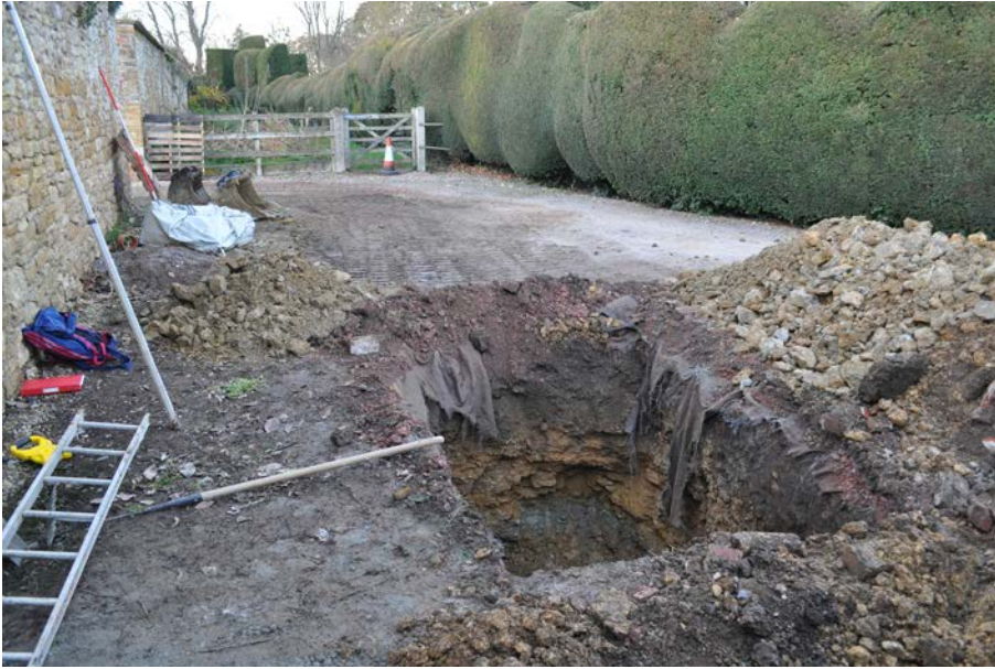
Plate 4: Trench 2 after excavation, looking north.
