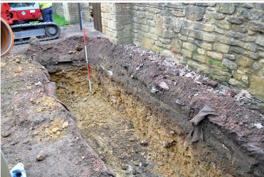
Plate 3: Trench 3 after excavation, viewed from west. 2m scale.
