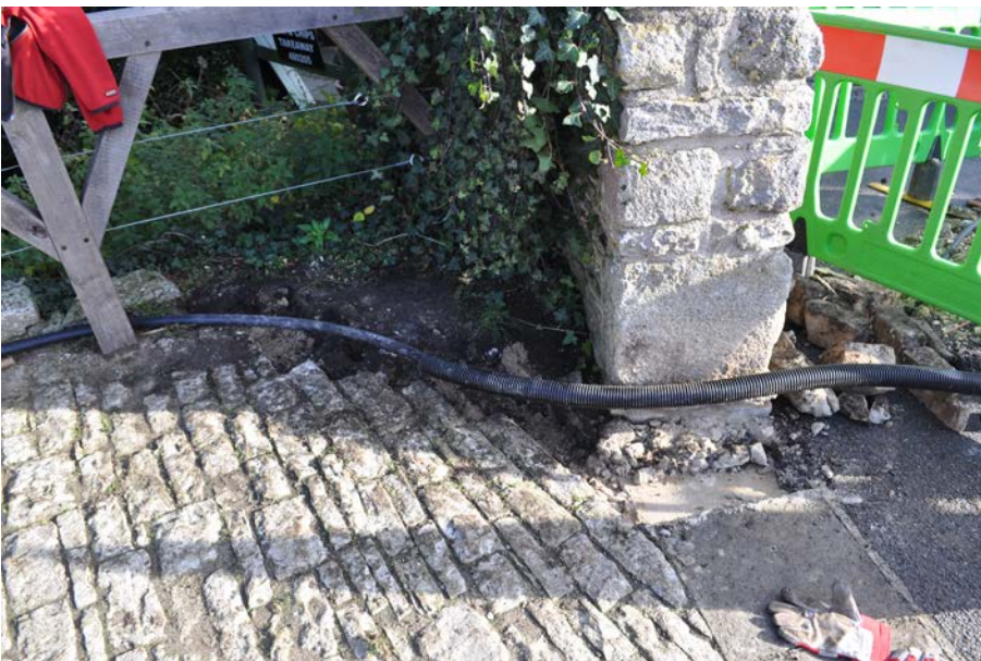
Plate 8: Trench 4 after excavation. View from west.
