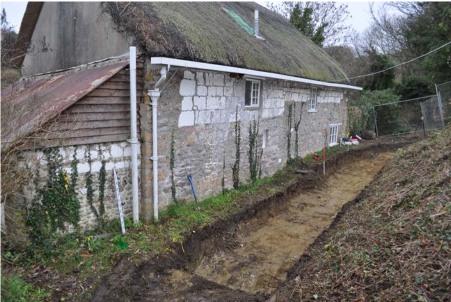
Plate 2: View of trench after excavation, viewed from south. 1m scale.
