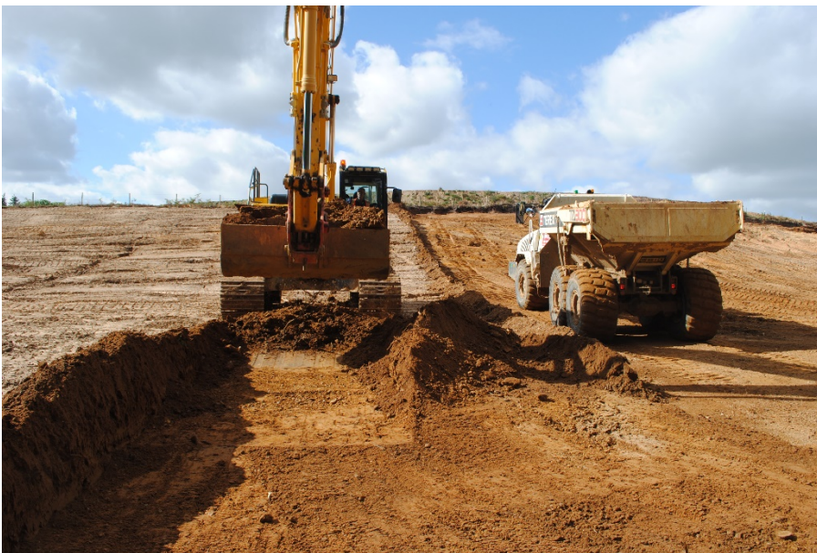
Plate 2: Stripping of subsoil/former ploughsoil. View from east.
