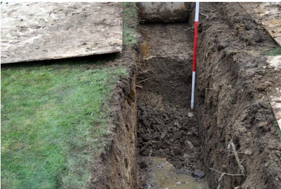
Plate 5: Ditch 110 to right and Robber Trench 108 on left side of new heat main trench, viewed from NNW. 2m scale.
