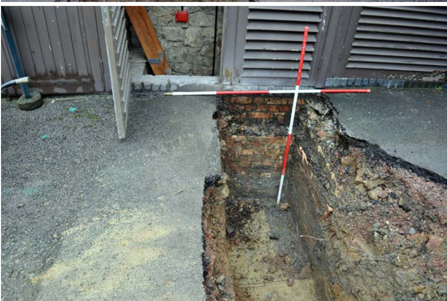
Plate 9: Walls of Strode House boiler room 120, in construction trench 121, viewed from W. 2m scales.
