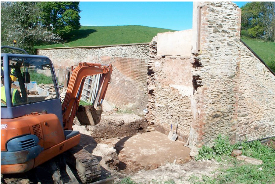
Plate 2: View of works on Room 1.
