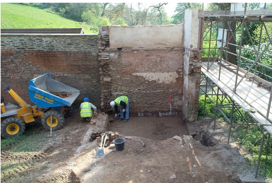
Plate 3: View along Stock House towards the east.
