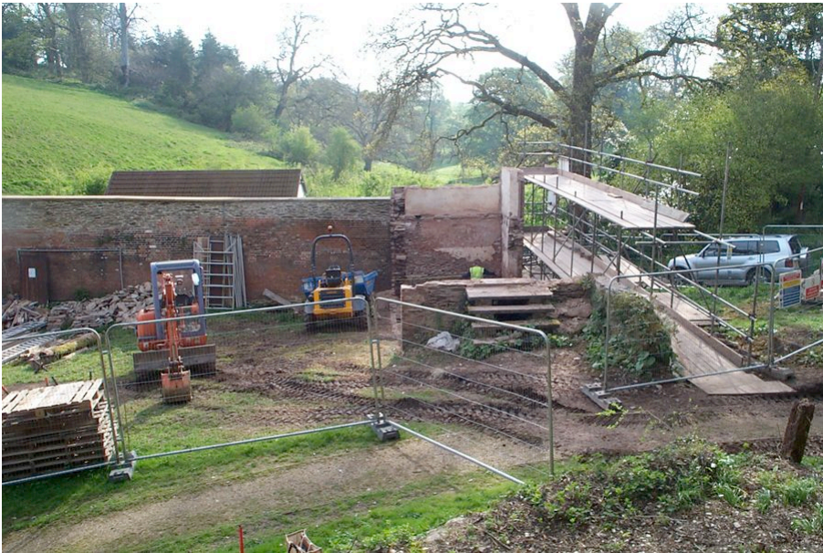
Plate 1: General view of site of stock house viewed from west.
