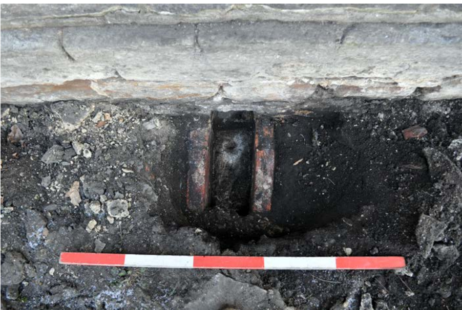
Plate 12: Drain 115 with concrete 117 at end of drain. View from north. 1m scale.
