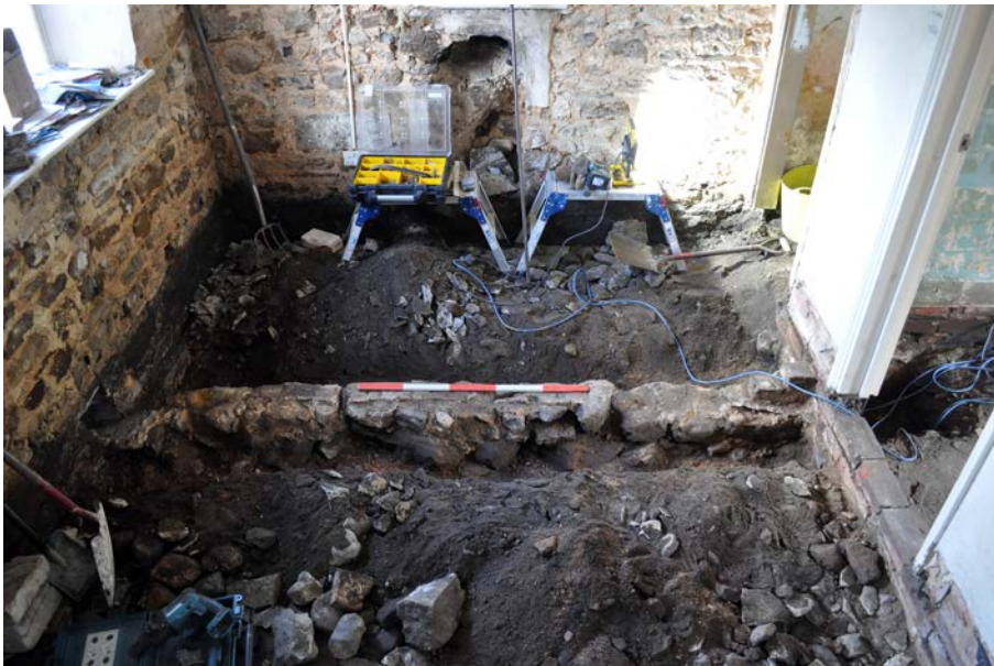
Plate 5: North Room looking east with exposed Structure 111. 1m scale.
