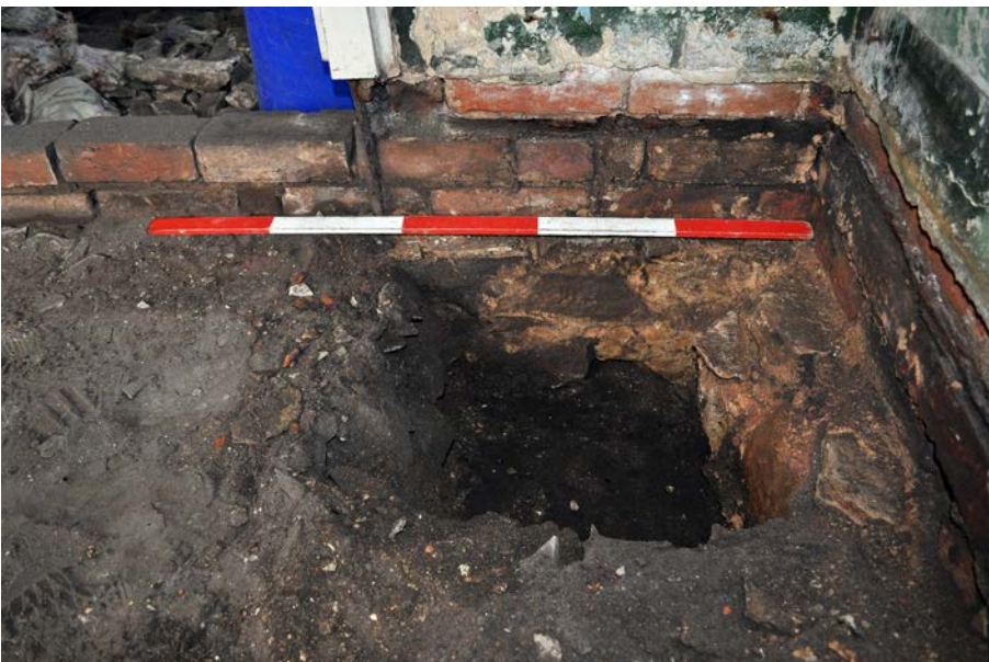
Plate 2: Sondage dug in NE corner of South Room showing mortared stone footings 104 and brick footings 114 above, looking north. 1m scale.
