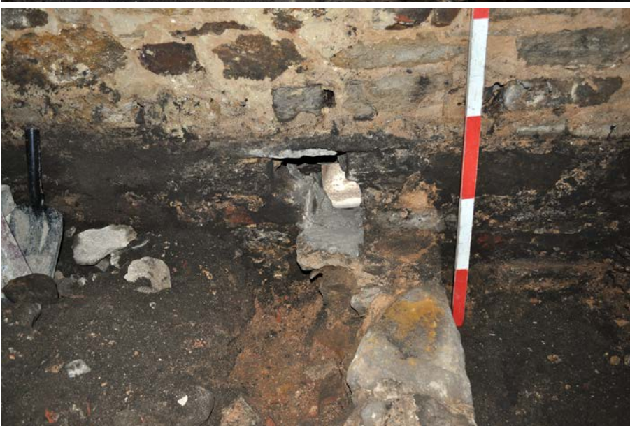
Plate 9: Drain 115 through north external wall and Structure 111 to right with vertical line scored in north wall just visible to left of scale. 1m scale.
