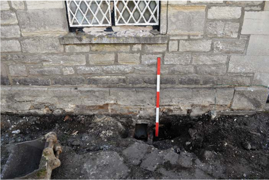
Plate 10: External view of drain 115. View from north. 1m scale.
