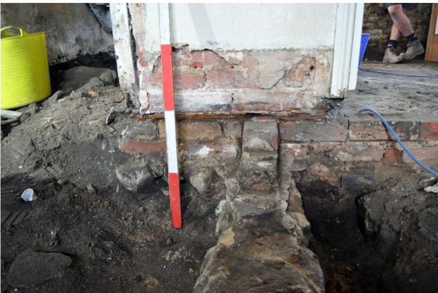
Plate 8: Detail of relationship between structure 111 and internal wall between North and South Rooms. 1m scale.
