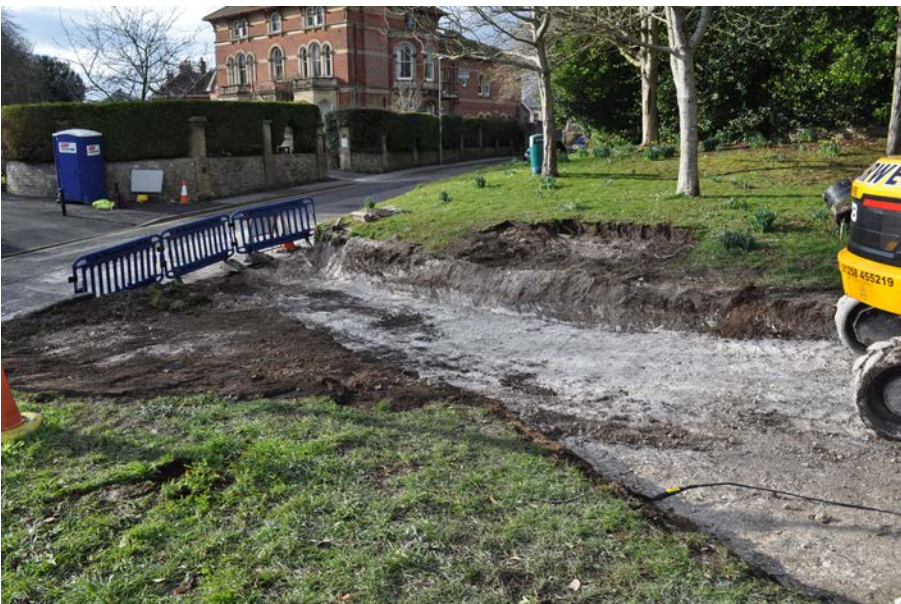
Plate 2: View of trench during reprofiling of the path, looking west.
