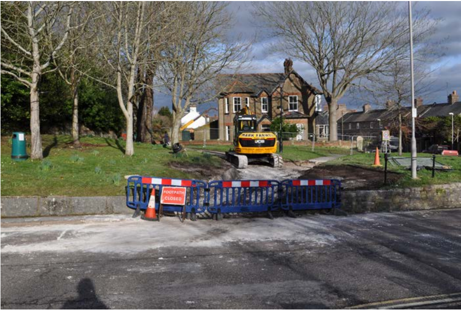
Plate 1: General view of site looking across Icen Way from the west.
