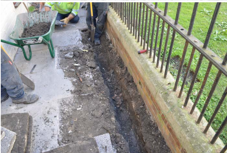
Plate 3: Group of broken skull fragments overlying electricity cable in trench, looking west.
