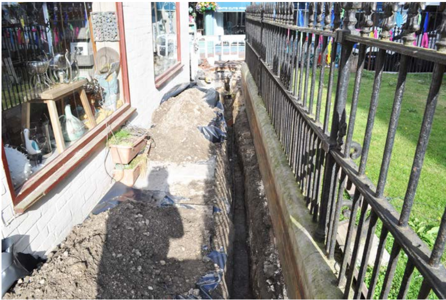
Plate 1: General view of trench looking west towards St Mary Street.
