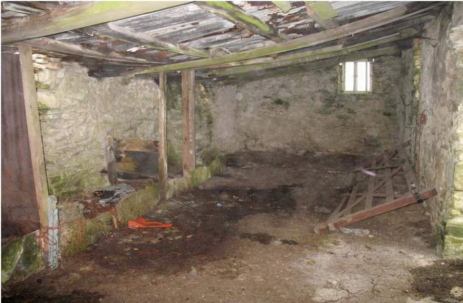
Plate 5: Building A – interior view.
