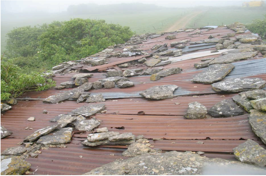
Plate 4: Building A – exterior view of roof.
