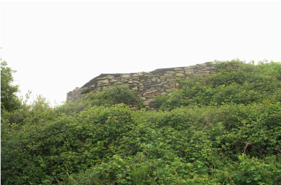
Plate 8: Building B – exterior view of northwest corner.
