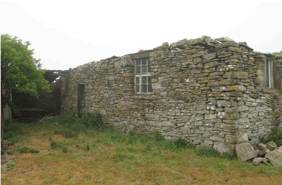
Plate 2: Building A – exterior view of west wall.
