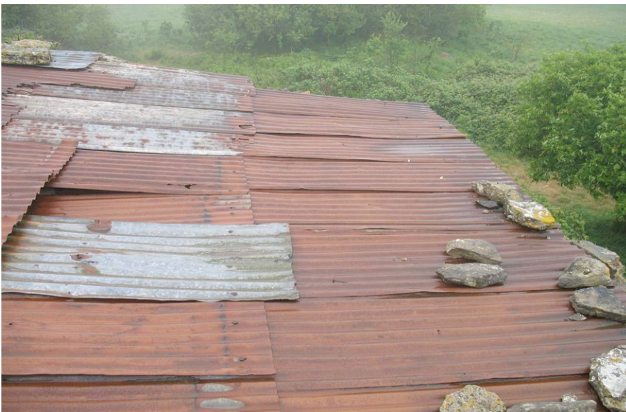
Plate 9: Building B – exterior view of roof.
