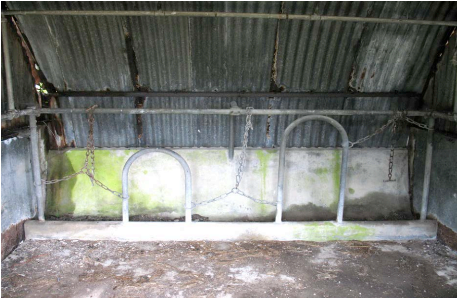
Plate 17: Building D – interior view.
