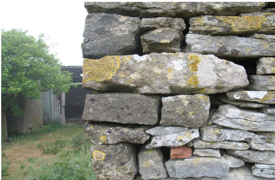
Plate 27: W1 – pair of wedge pits on underside of stone (Figure 3).
