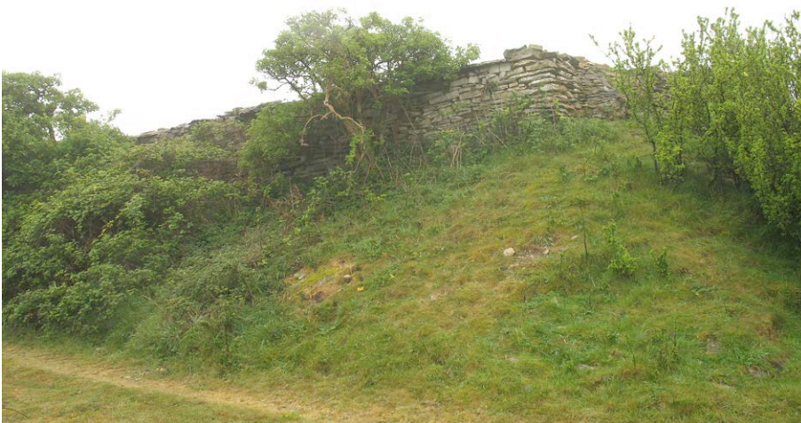
Plate 3: Building A – exterior view of northeast corner.
