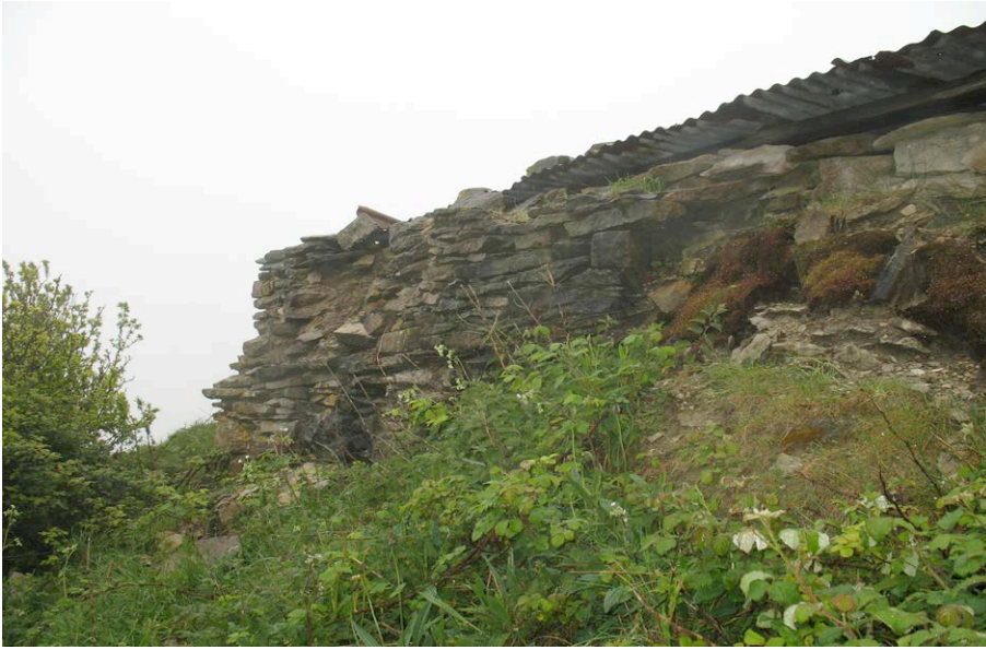
Plate 7: Building B – exterior view of north wall.
