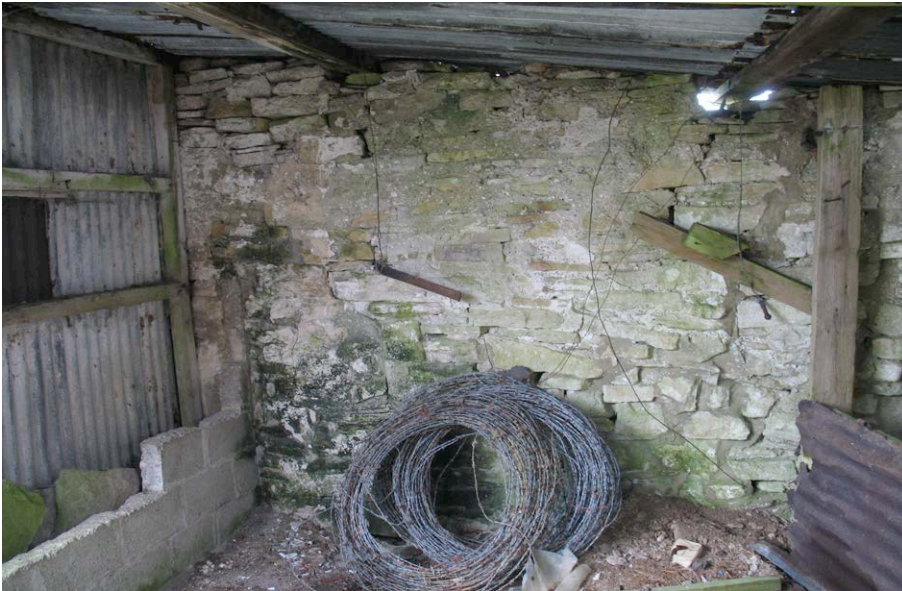
Plate 11: Building B – interior of west wall.
