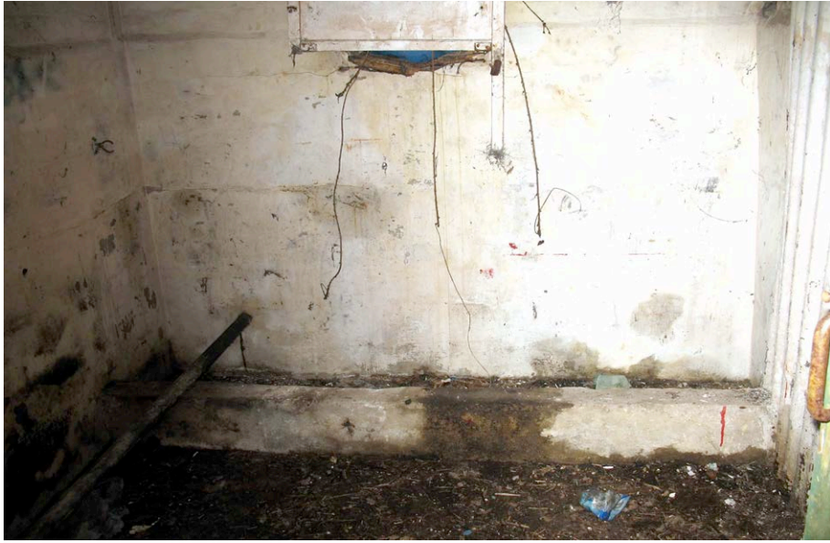
Plate 19: Building E – interior view.
