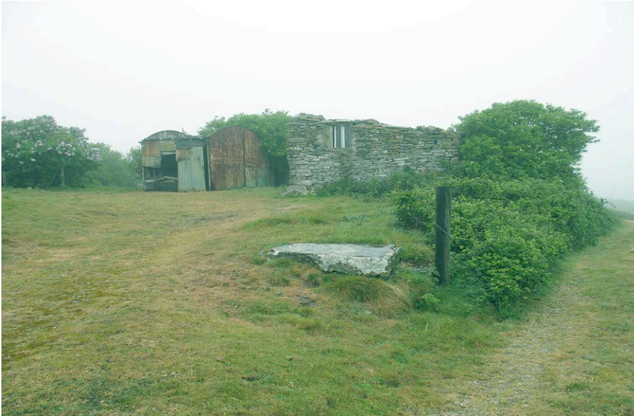
Plate 22: View of loading platform from southeast.
