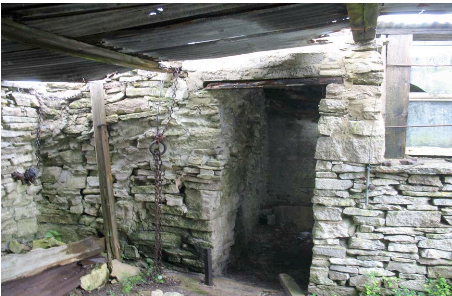
Plate 6: Building A – doorway leading from Building B.
