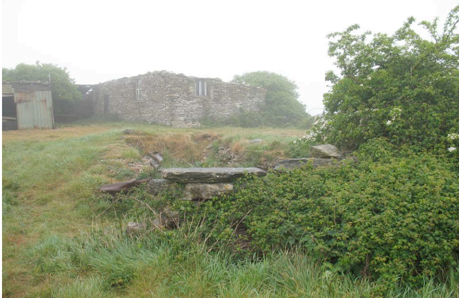
Plate 20: Structure F – view from south.
