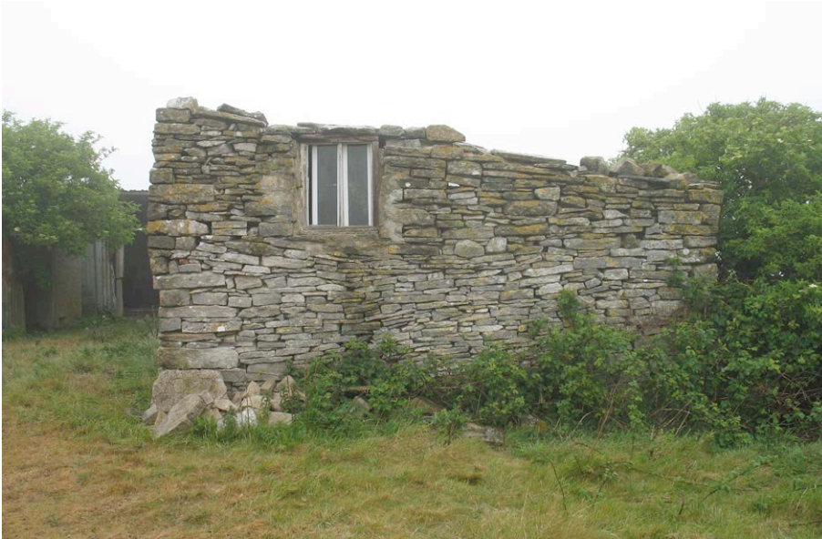
Plate 1: Building A – exterior view of south wall.
