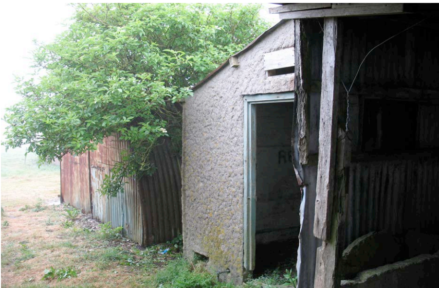
Plate 18: Building E – view from northeast.
