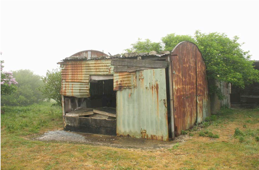
Plate 16: Building D – view from the southeast.
