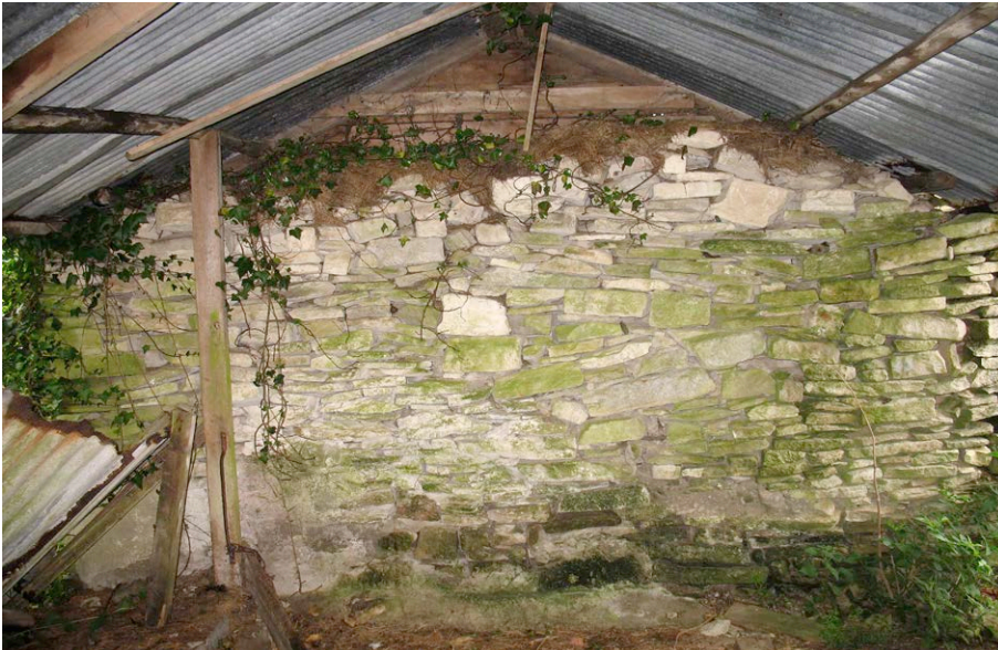
Plate 14: Building C – interior view of north wall.
