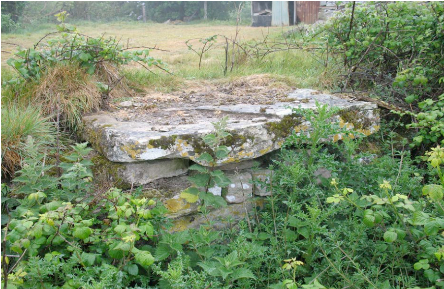
Plate 23: Detail of loading platform.
