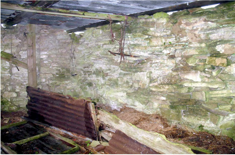
Plate 10: Building B – interior of north wall.
