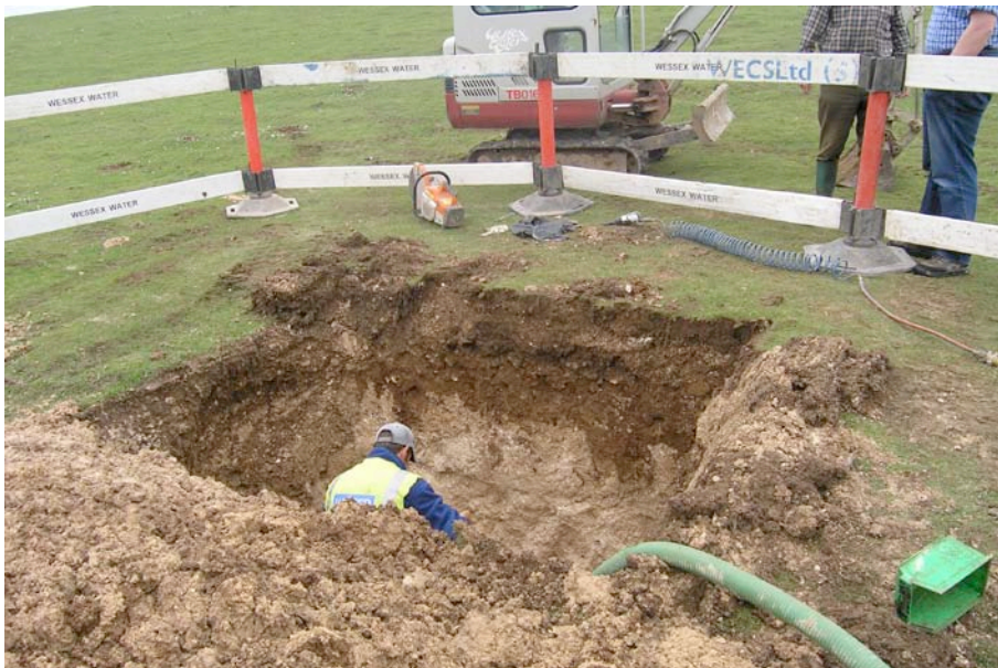
Plate 5: View of north-facing section of trench.
