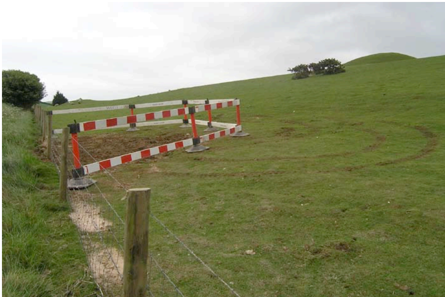
Plate 8: View looking east towards the Scheduled Area after backfilling.
