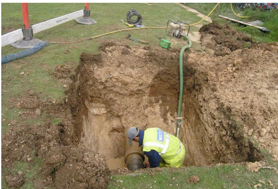
Plate 6: View of east-facing section of trench, showing pipe trench.
