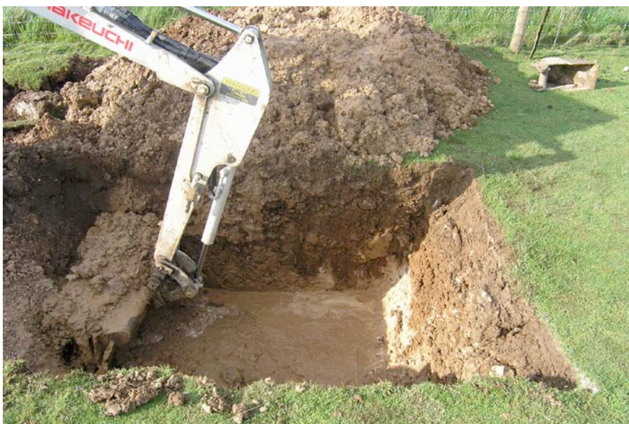
Plate 2: View of trench during excavation – from south.
