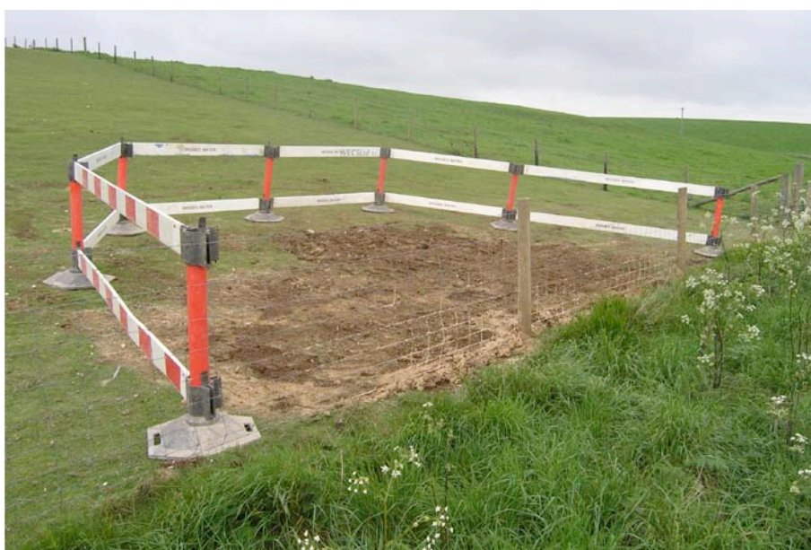
Plate 8: The site after backfilling, looking southwest.
