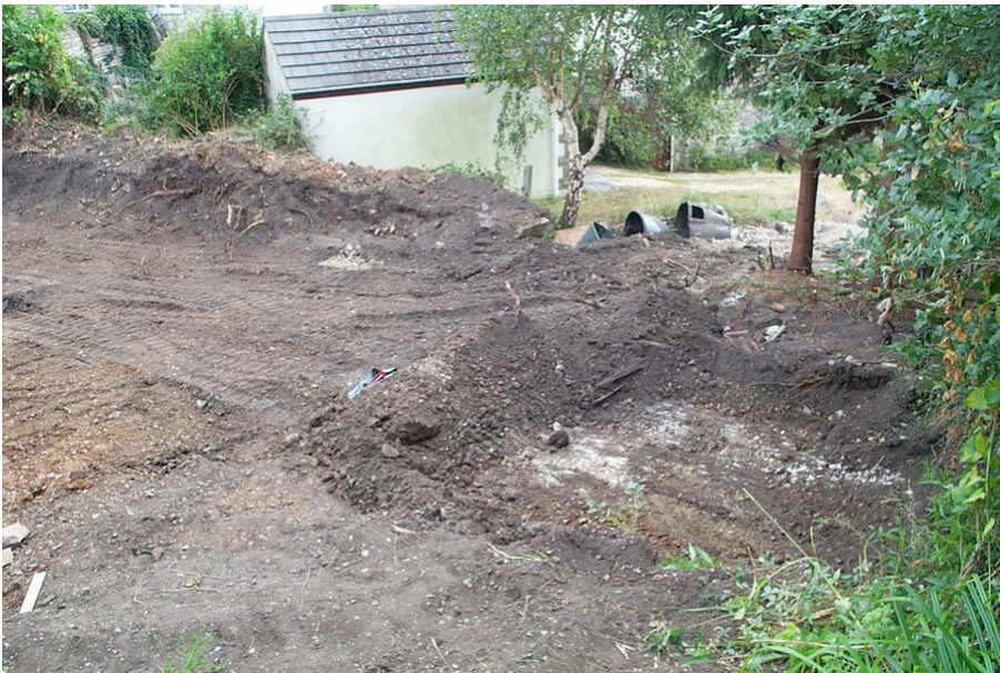
Plate 2: Southern end of site after topsoil stripping and levelling.
