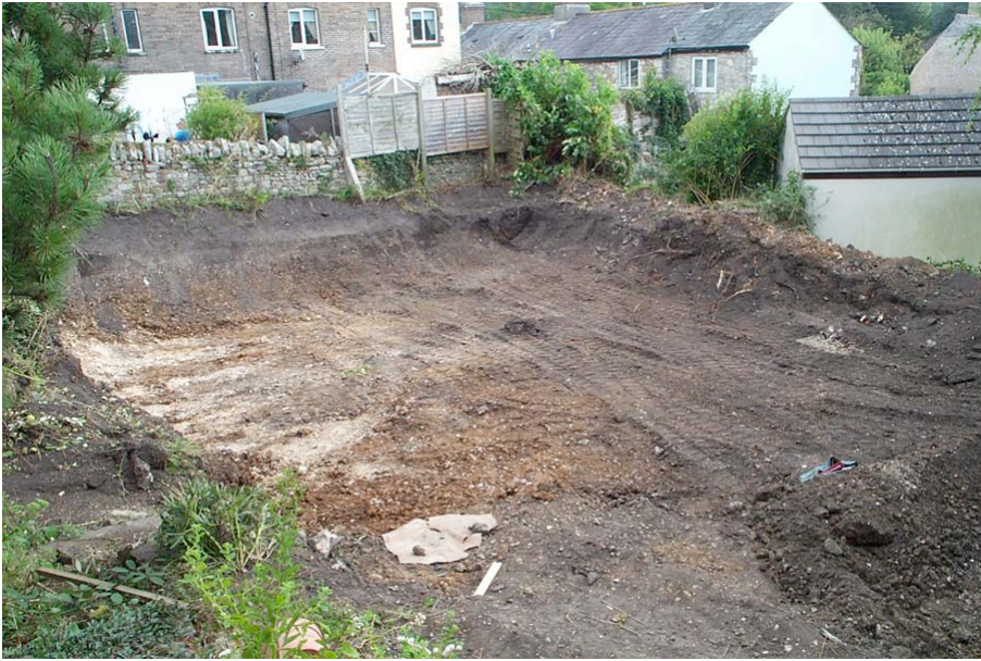
Plate 1: Northern end of site after topsoil stripping and levelling.
