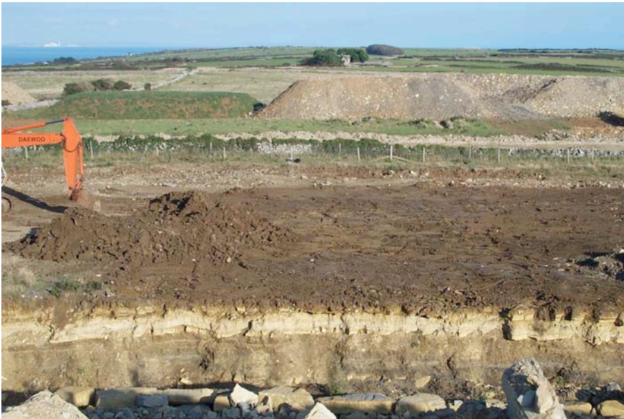
Plate 2: View of northern half of stripped area, looking east.
