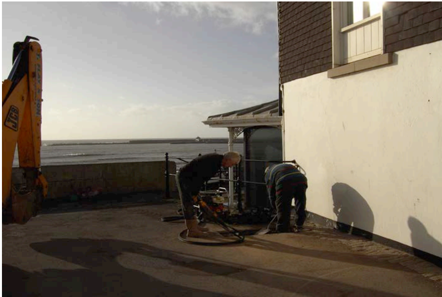
Plate 10: Test Pit 2 – location shot.
