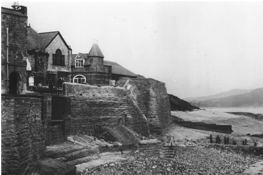
Plate 7: Postcard from 1930 showing cottages in process of being demolished.
