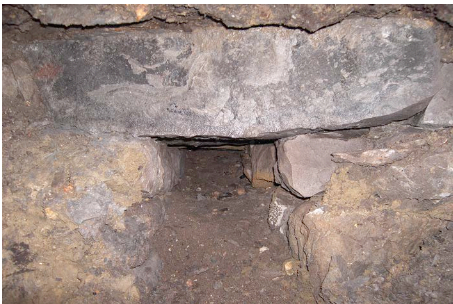
Plate 12: Test Pit 2 – southern elevation of culvert.
