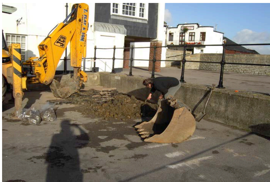
Plate 13: Test pit 4 – location shot.
