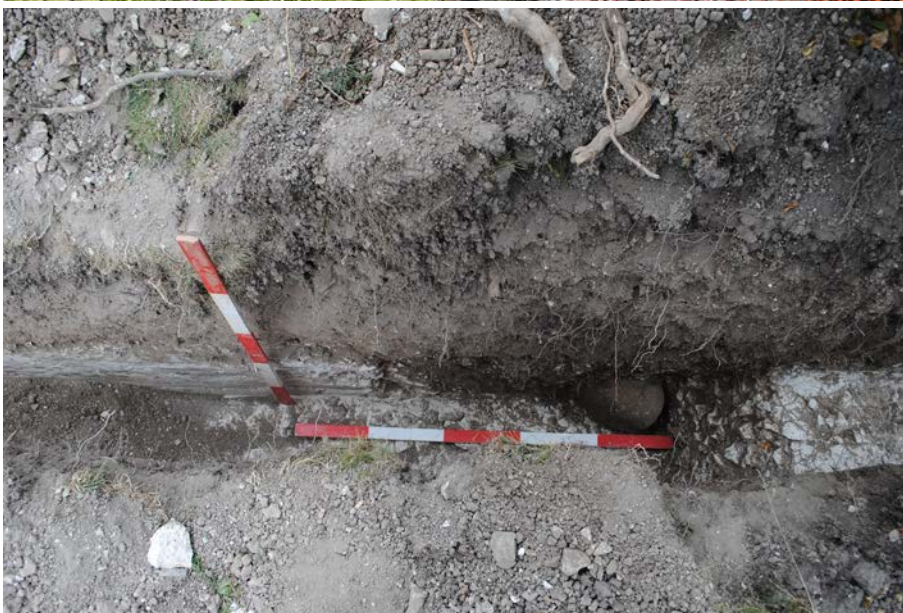
Plate 3: Work on the service trench through the garden north
