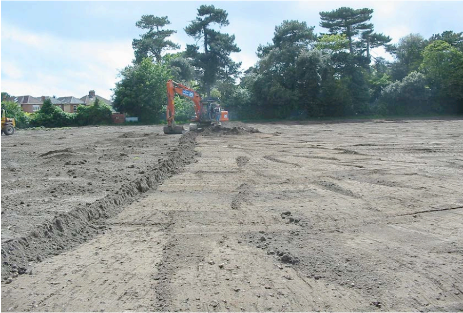
Plate 1: General view during stripping, looking southwest.
