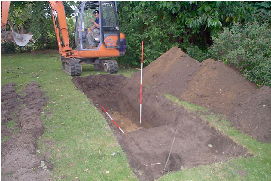
Plate 8: Trench 3 viewed from west.
