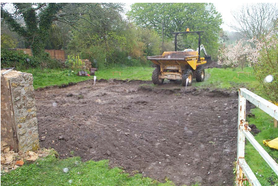
Plate 3: Stripped area, looking northeast.
