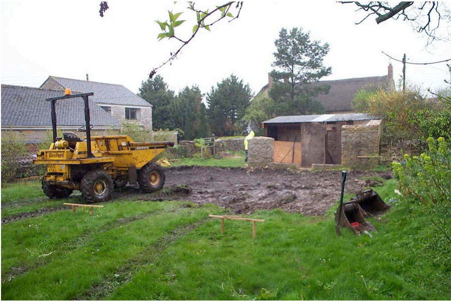
Plate 1: General view of site from northeast.
