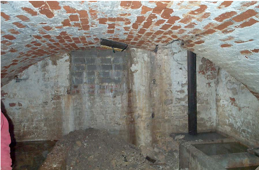
Plate 4: West end of northern cellar.
