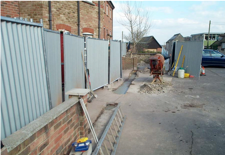
Plate 2: East end of the footings trench, looking east.
