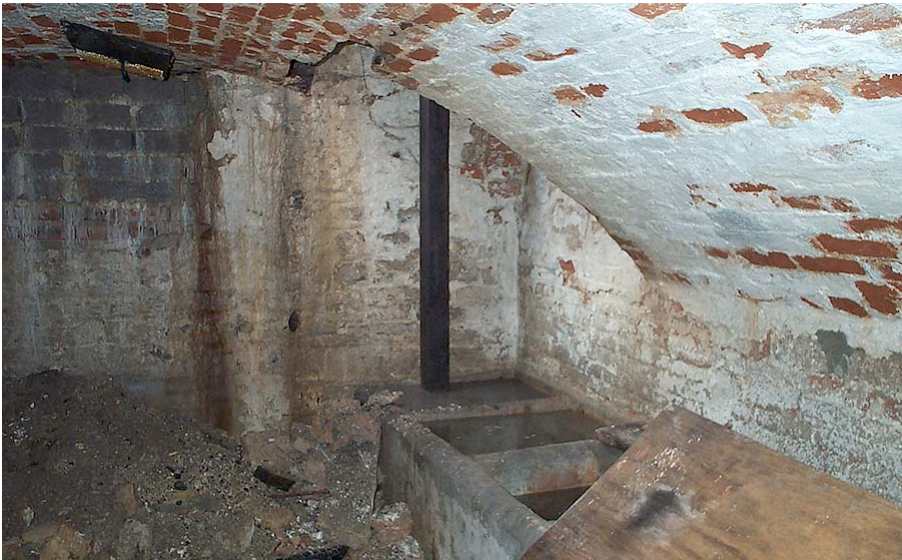
Plate 6: Vats along northern side of northern cellar, looking west.
