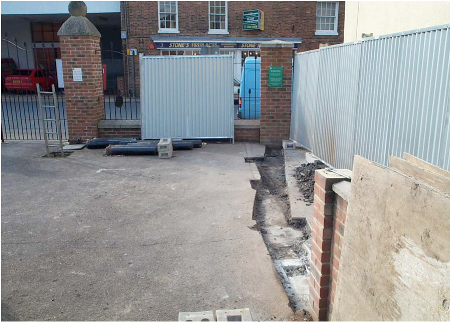
Plate 1: Western part of wall footings trench, looking west towards the road.
