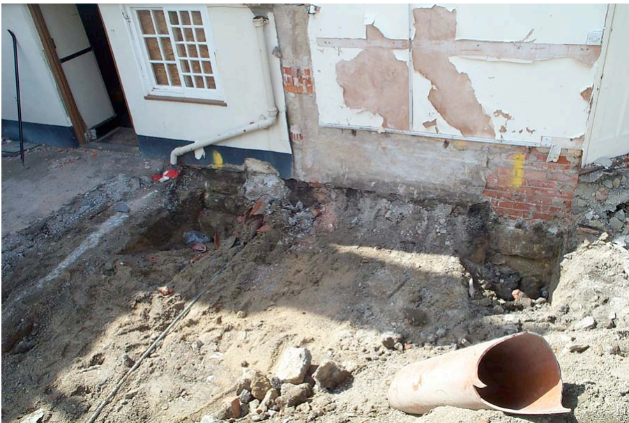
Plate 5: Test Pits 2 and 3 showing stone footings to building.
