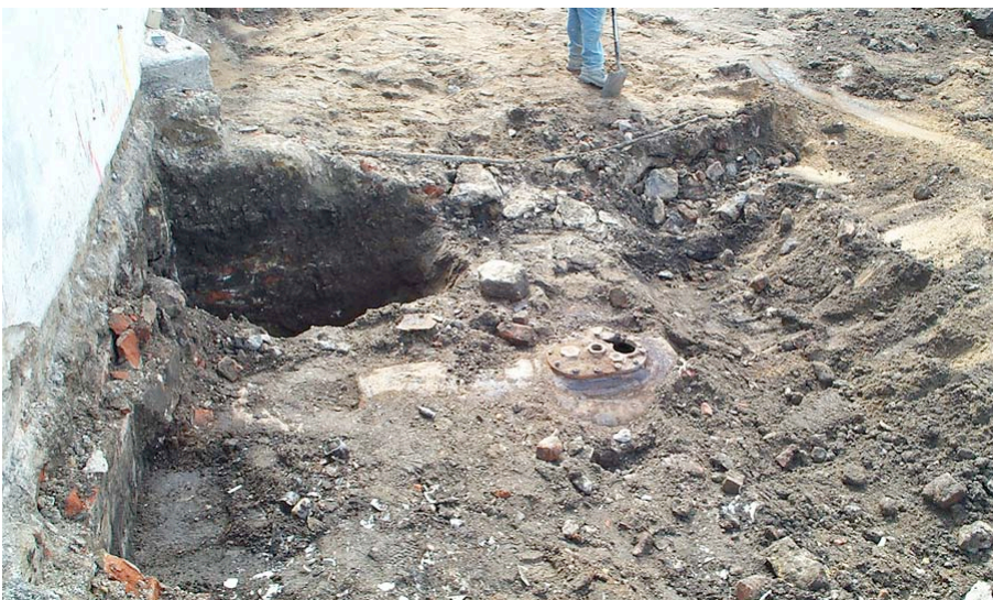
Plate 6: Test Pit 8 with fuel tank in foreground, from north.
