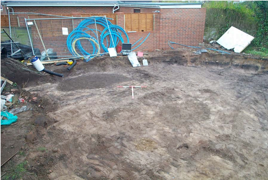
Plate 1: General view of stripped area looking northeast.
