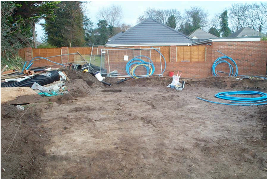
Plate 2: View of stripped area after excavation, looking north.
