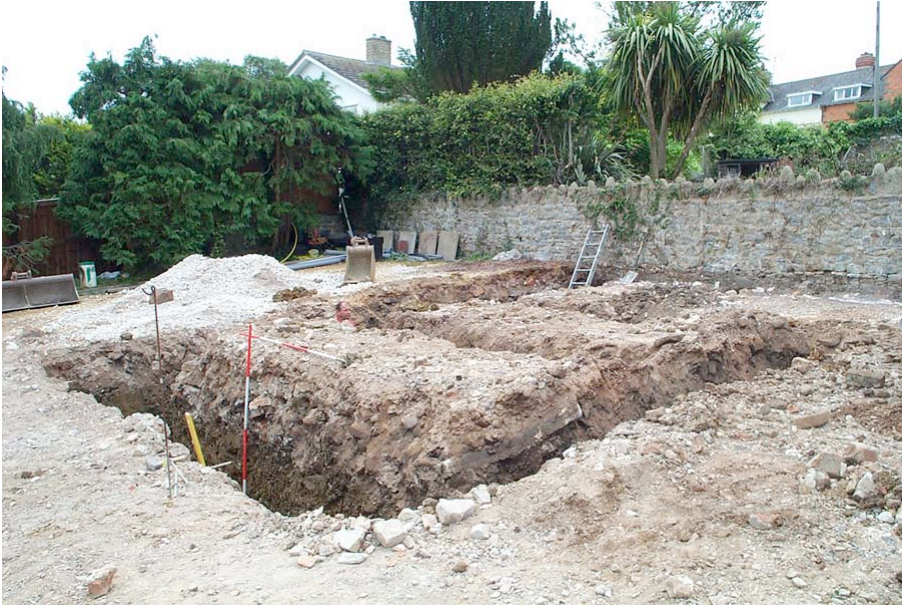
Plate 1: General view of footings trenches from northeast.
