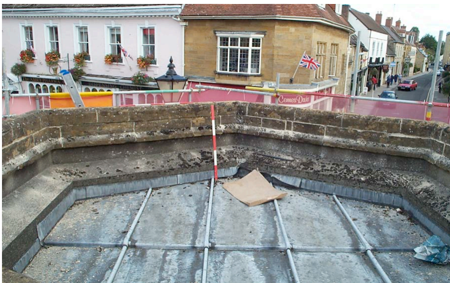
Plate 6: Lead roof, looking east.
