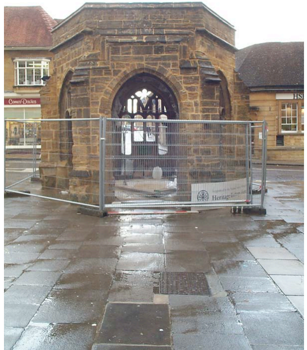
Plate 10: West front, after repointing.
