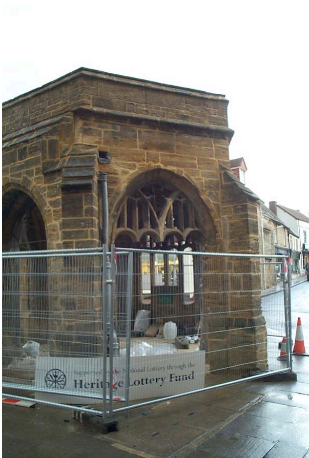
Plate 11: Southwest front, after repointing.
