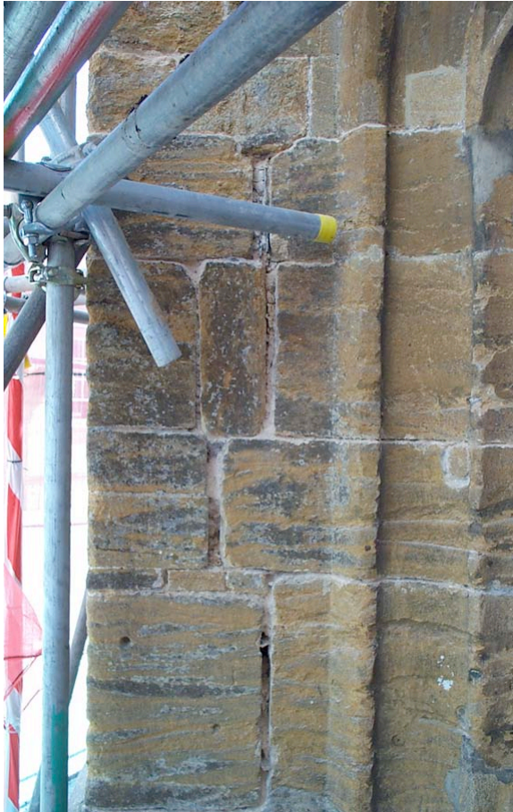
Plate 1: Detail of north face of NE buttress showing differences in mortar and slate packing.
