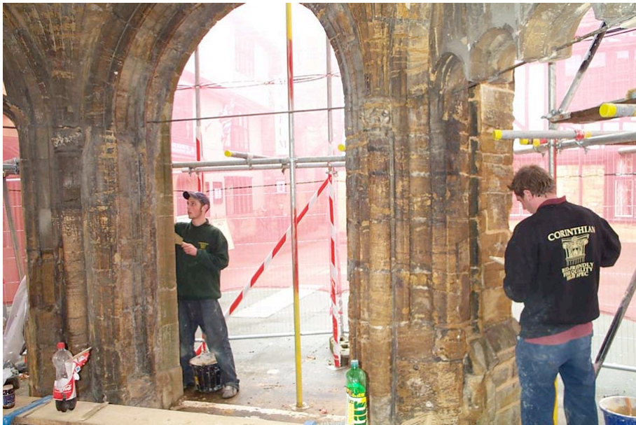
Plate 8: Repointing the structure.
