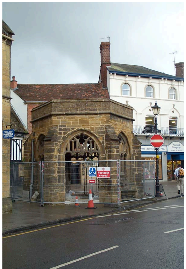
Plate 12: Southeast front, after repointing.
