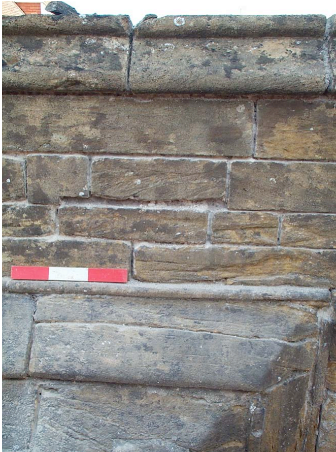
Plate 1: Detail of north face of NE buttress showing differences in mortar and slate packing.
