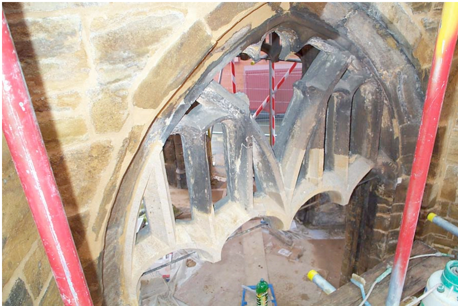
Plate 5: Detail of tracery in NW front after repair of stonework.
