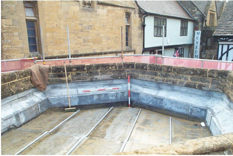
Plate 7: Lead roof after repair work completed, looking west.
