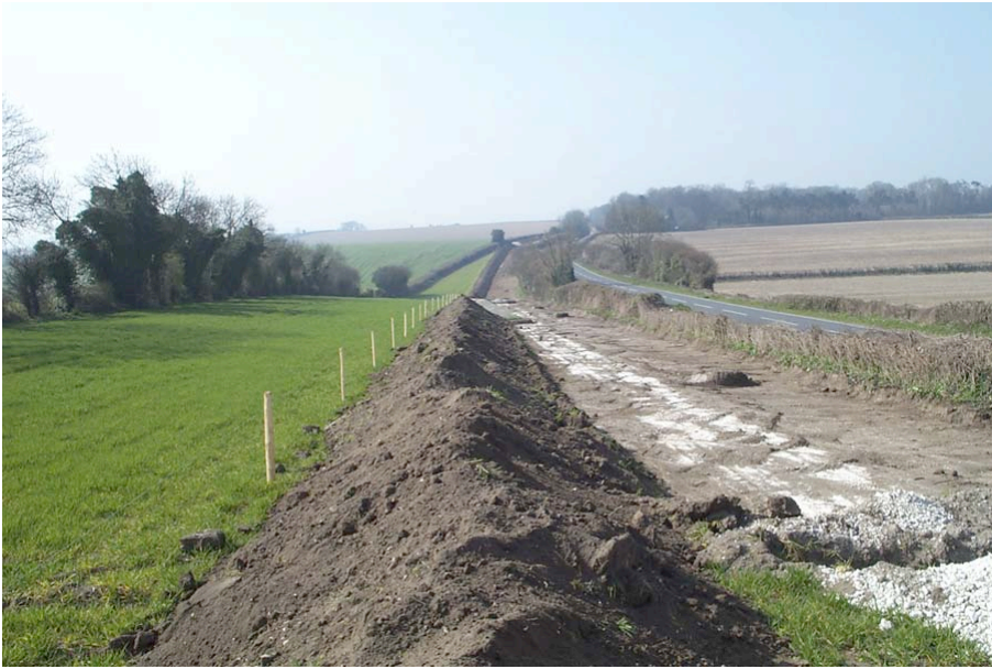
Plate 1: View along easement looking southwest towards Longthorns Wood.
