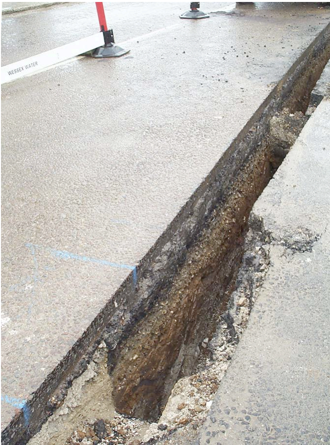
Plate 2: View of north-facing section of pipe trench.
