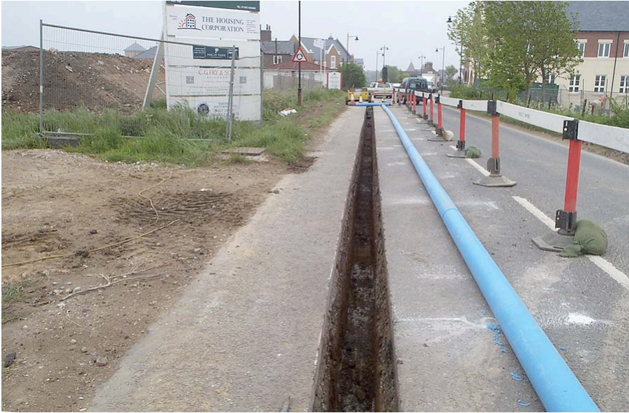
Plate 1: General view along pipe trench from the west.
