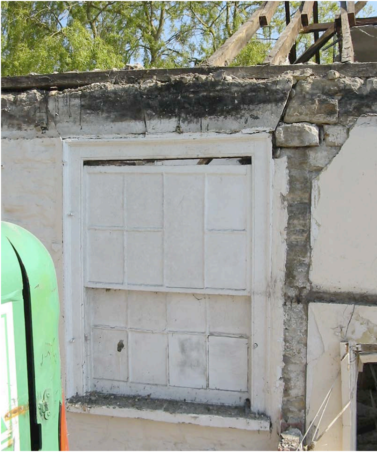
Plate 5: Detail of surviving window in north elevation.
