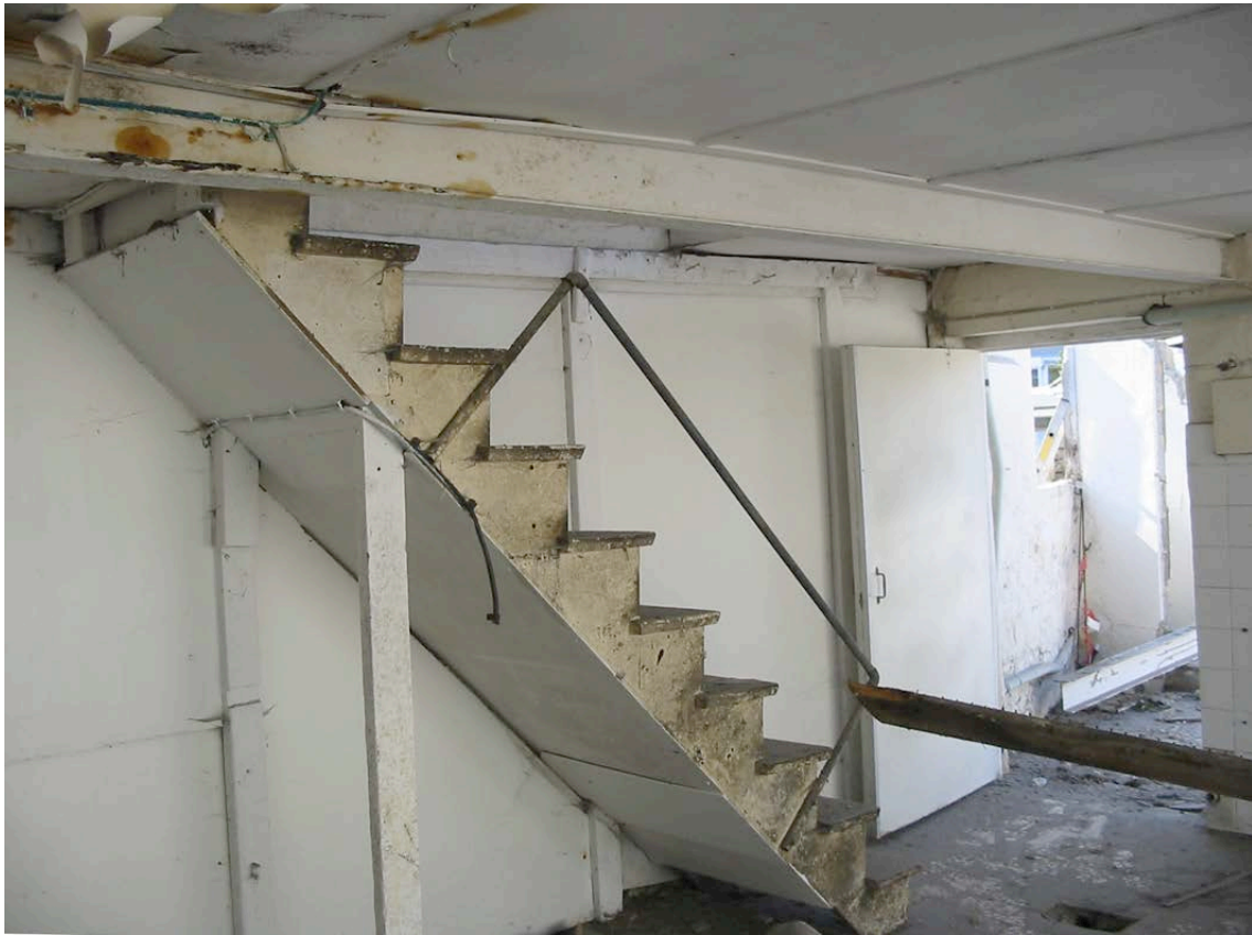
Plate 19: Detail of stairs to gallery
