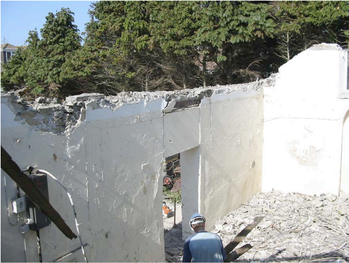
Plate 13: North internal wall from gallery
