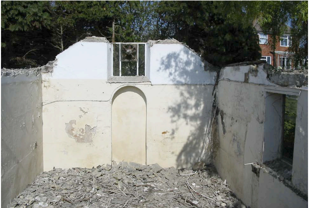
Plate 11: View of east end of interior of chapel
