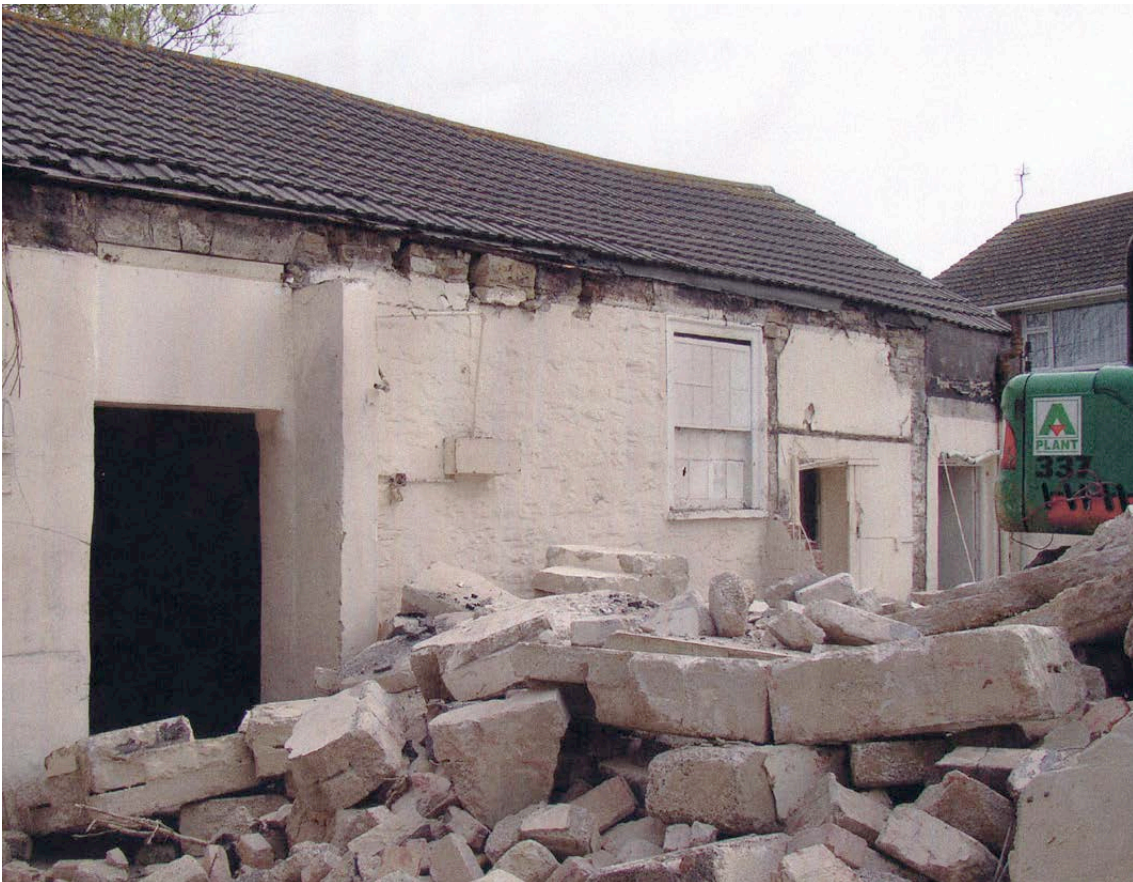
Plate 2: West end of north elevation (photo by Betterment Properties (Weymouth) Ltd)
