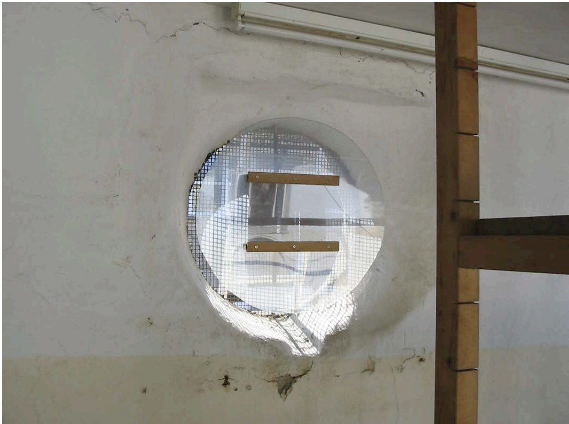
Plate 15: Detail of window in west gable
