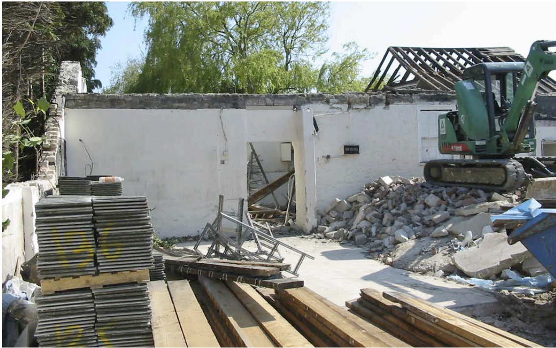
Plate 3: East end of north elevation after removal of the roof
