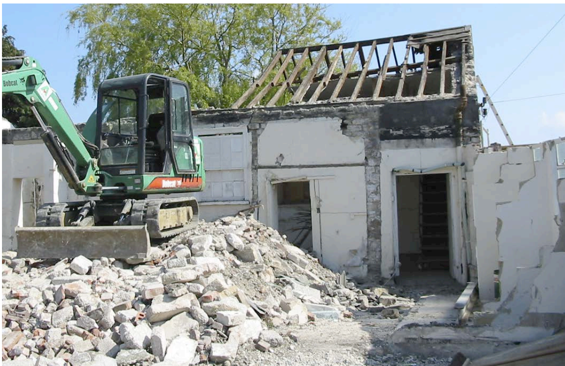
Plate 4: West end of North elevation during removal of roof.
