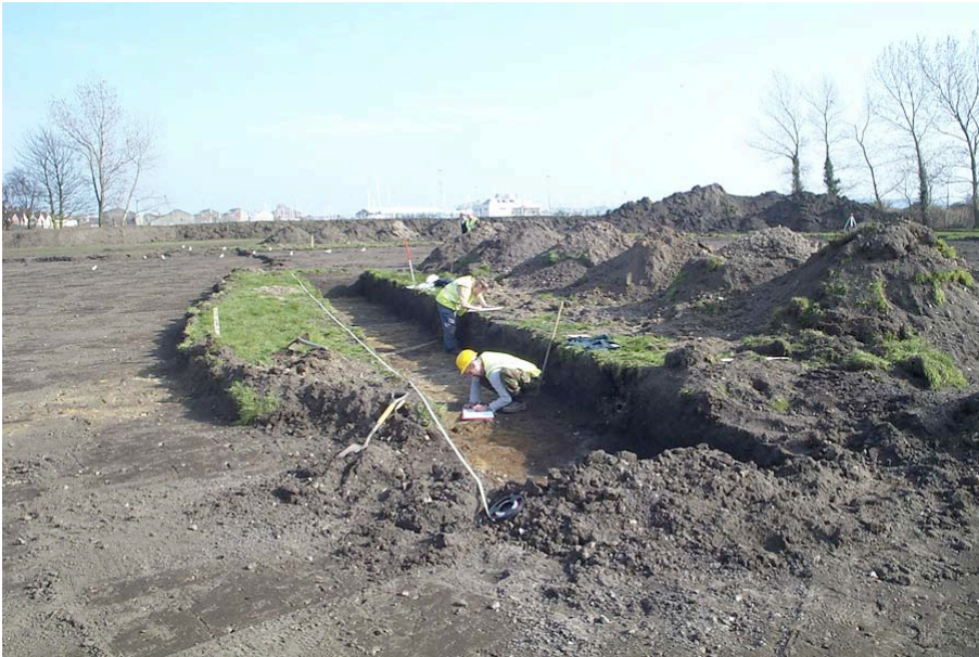
Plate 5: General view of Trench 5 from west.
