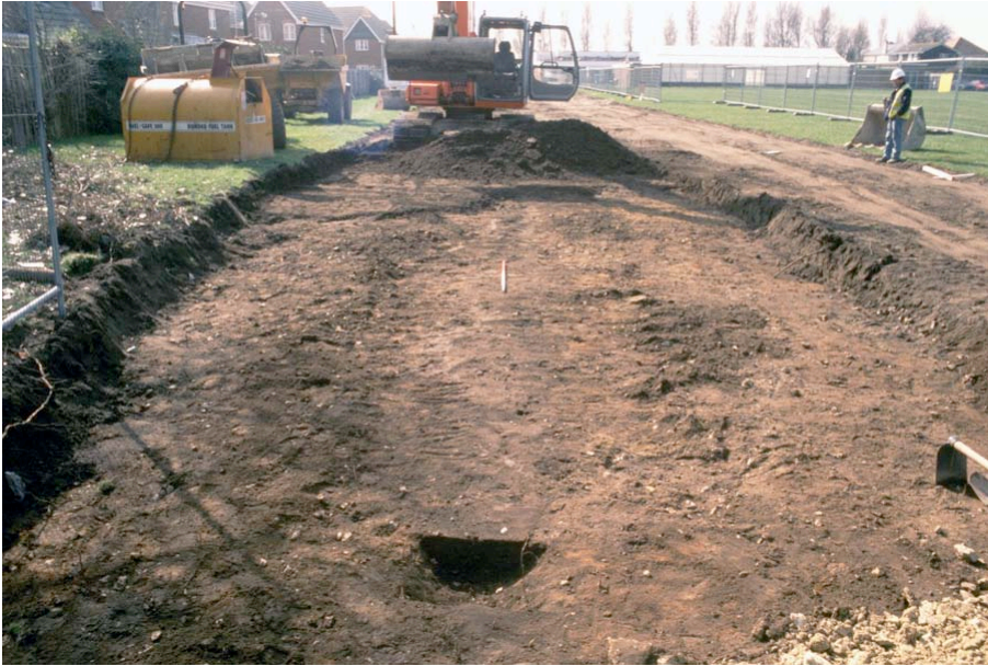
Plate 1: Trench 1 and Ditch 104, from north.
