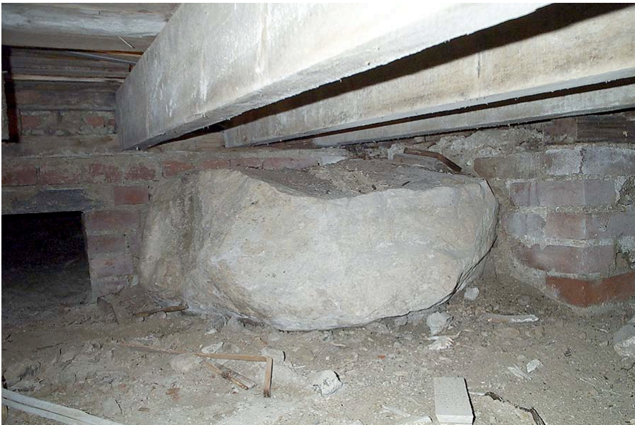
Plate 5: View below floor of large stone and sleeper walls built over, from north.
