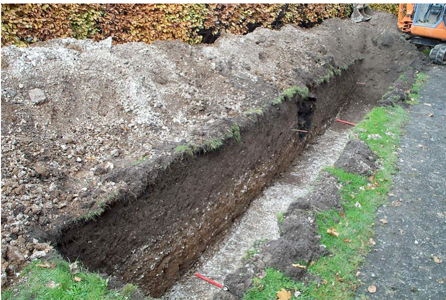
Plate 3: Trench 1 viewed from west.
