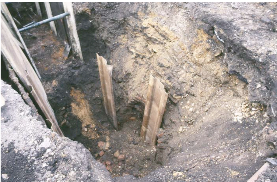
Plate 6: Ice well 8 after excavation of footings trench.
