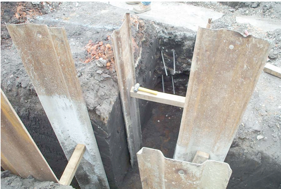
Plate 2: Typical view of deposits in footings trench, showing depth of layer 2.
