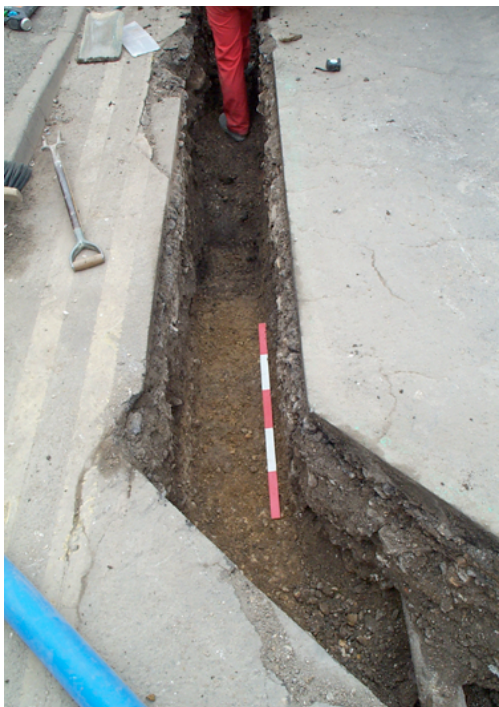
Plate 3: Roman road gravels in base of trench
