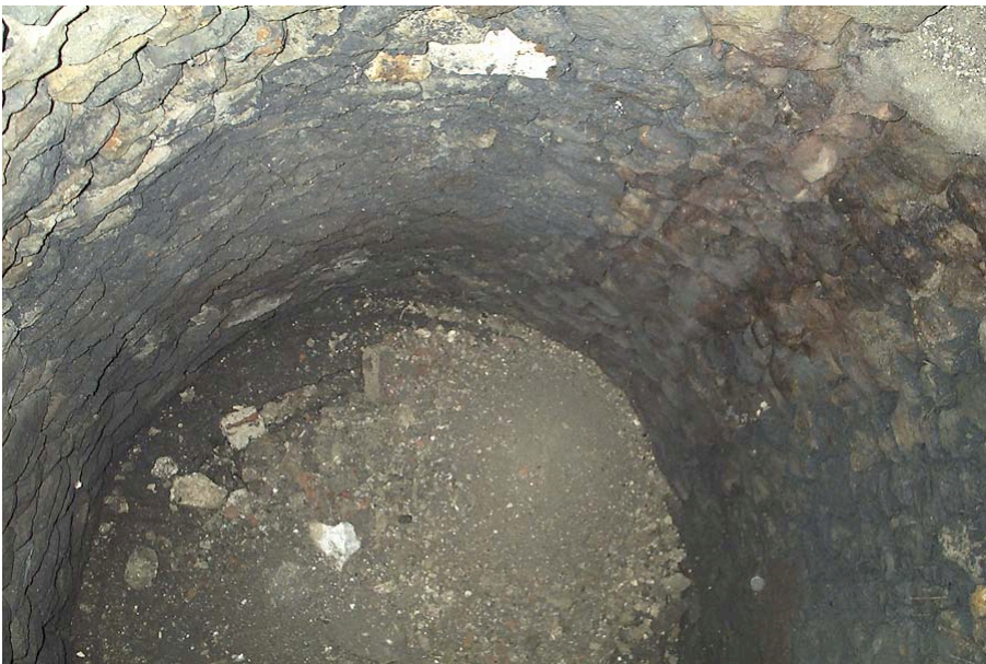
Plate 5: Detail of interior of ice well 704.
