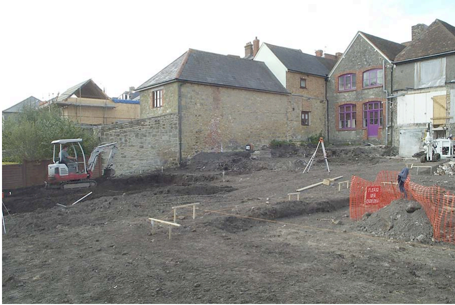
Plate 1: General view of site during groundworks, viewed from south east
