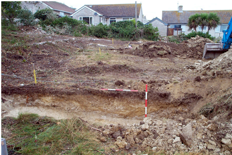
Plate 2: Trench 1 from southeast
