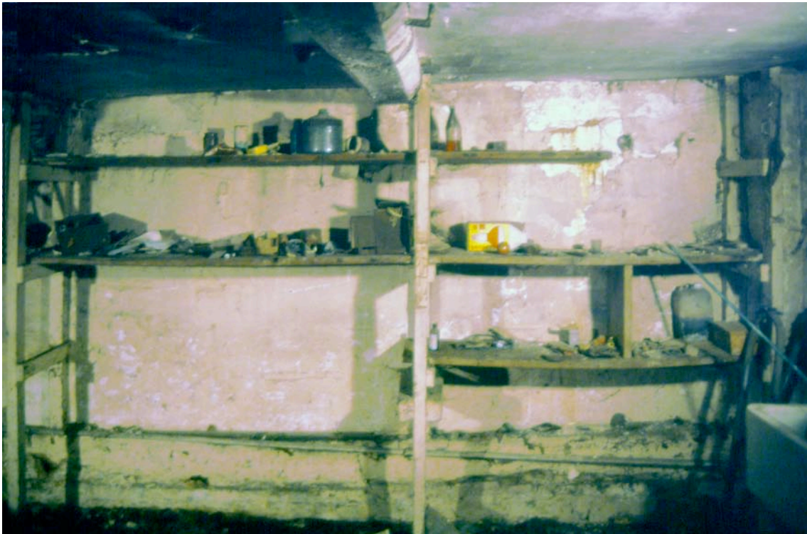
Plate 6: West wall, internal elevation
