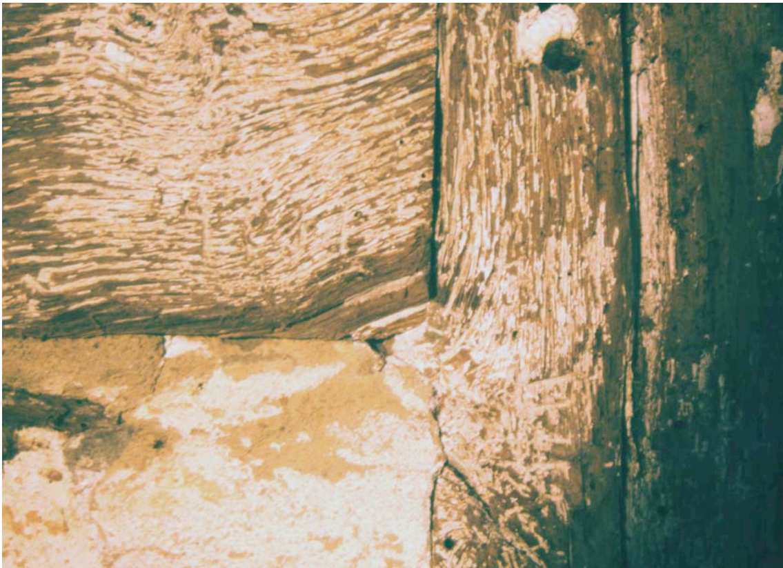
Plate 4: Detail of timber framing of west external elevation showing assembly marks
