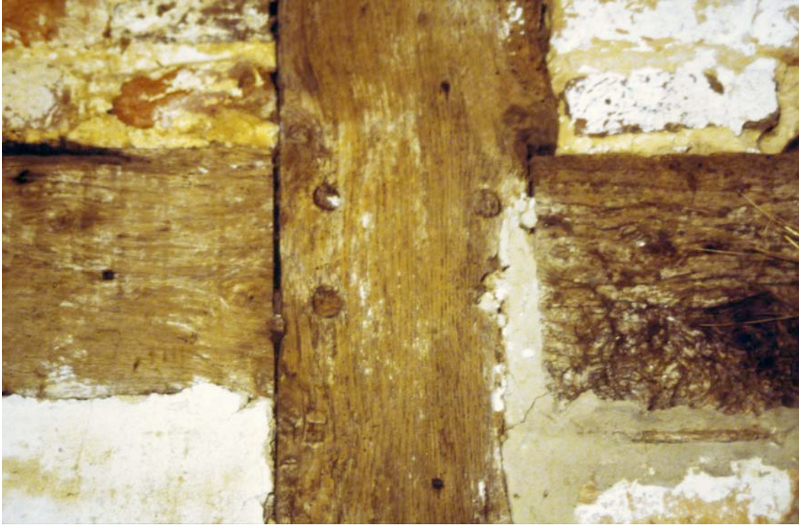
Plate 3: Detail of timber framing of west external elevation showing assembly marks.
