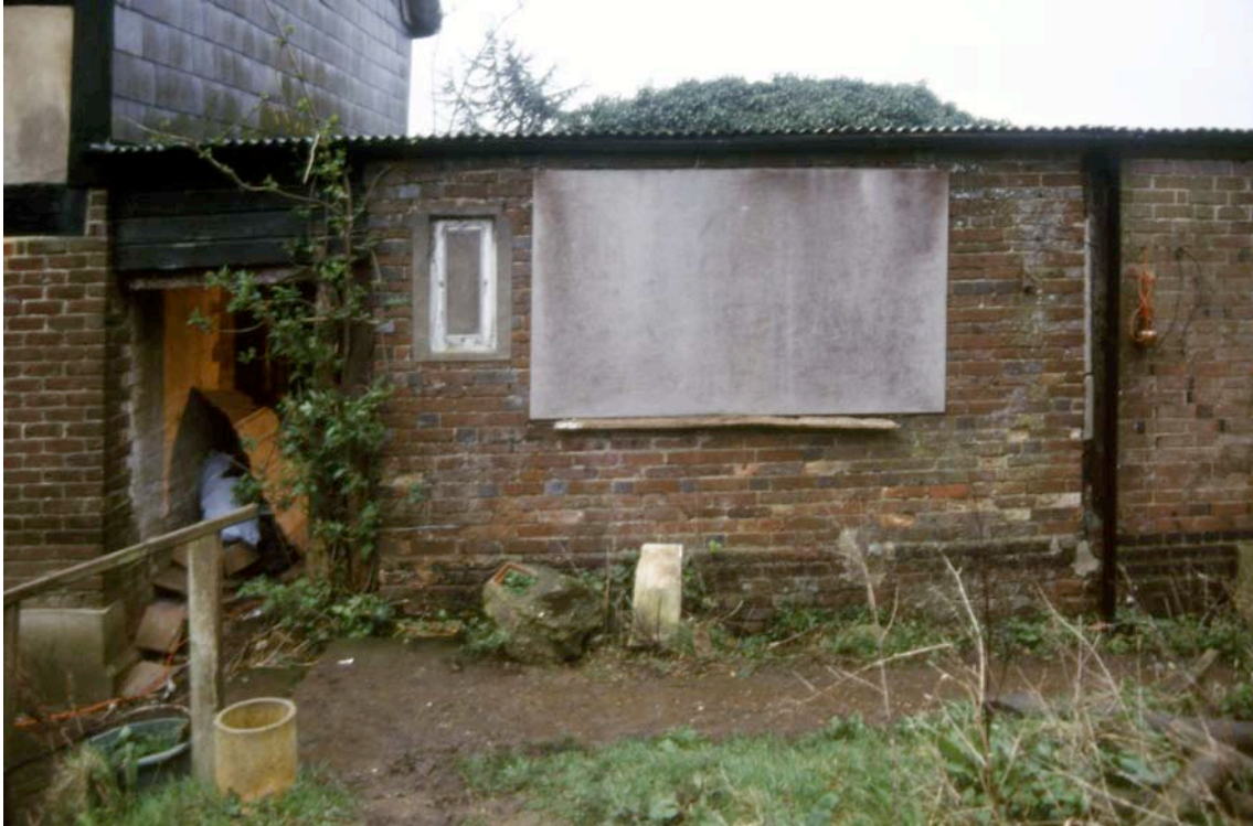
Plate 5: North wall, external elevation.
