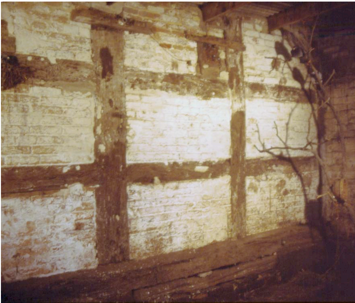
Plate 2: West wall, external elevation.
