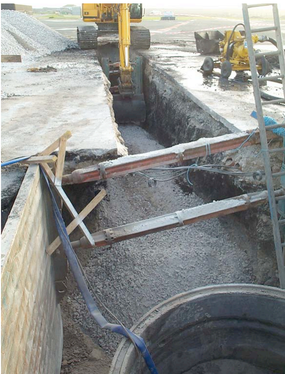
Plate 9: View looking southwest along Trench 2 during excavation.
