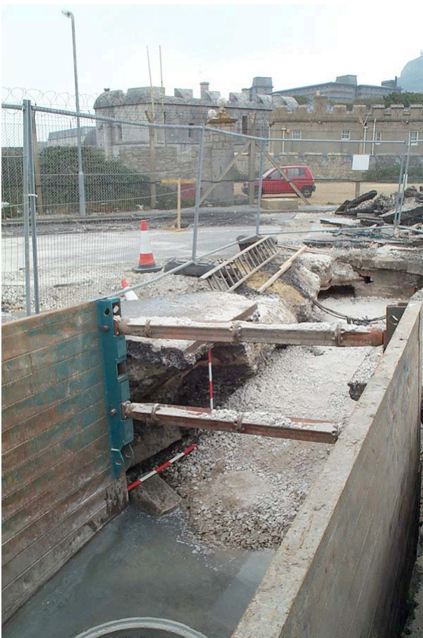
Plate 2: View looking east along Trench 1. Portland Castle in background. Large ashlar blocks visible just behind the shoring.
