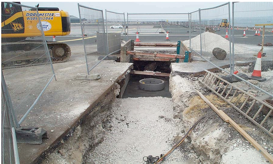
Plate 3: View northwest along Trench 1.
