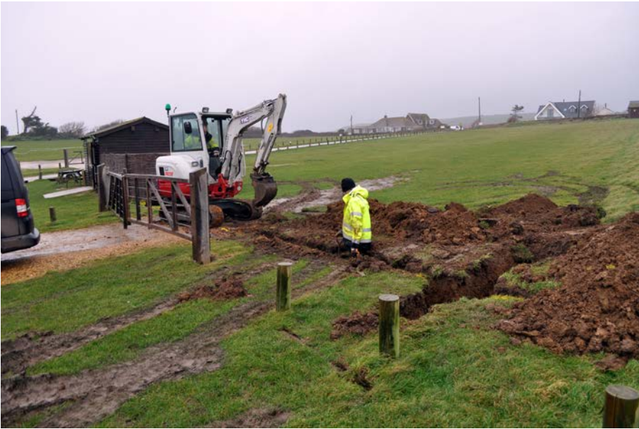
Plate 1: General view of trench during excavation, looking NW.
