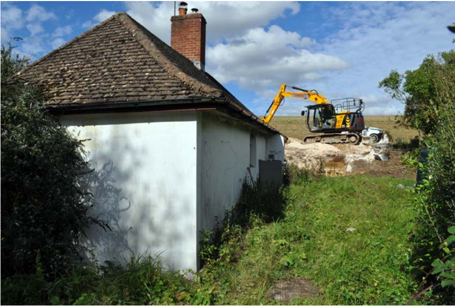
Plate 7: View of rear of N-S range showing cottage rising up slope.
