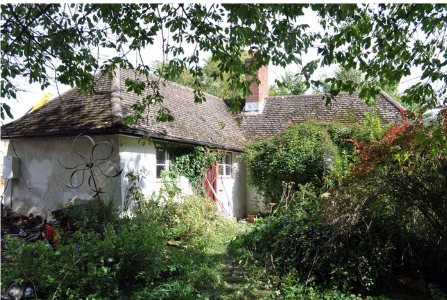
Plate 3: South and west external elevations of cottage, viewed from WSW.
