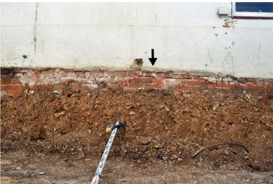
Plate 15: Detailed view of brick footings showing straight joint (arrowed).
