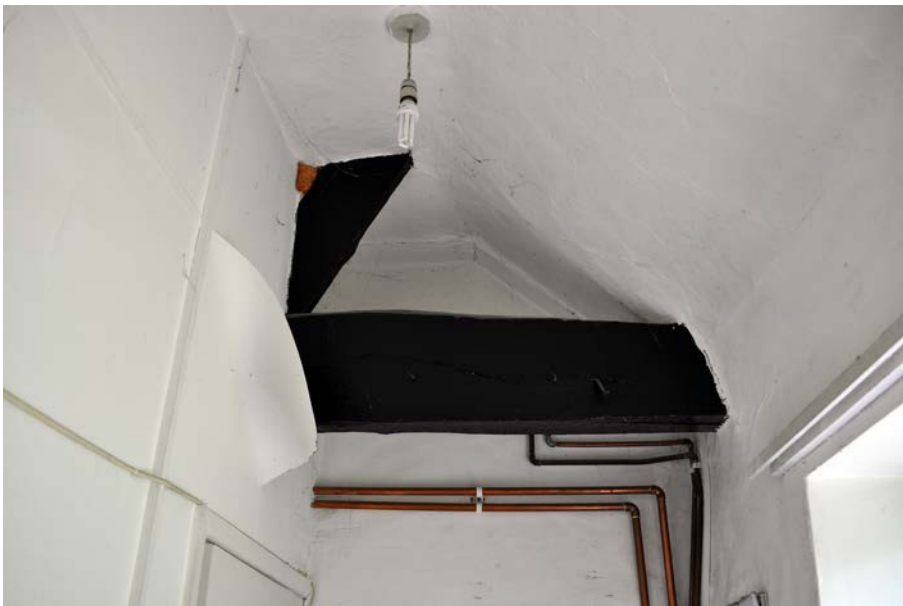
Plate 33: Exposed part of Truss 3 in Room 5.
