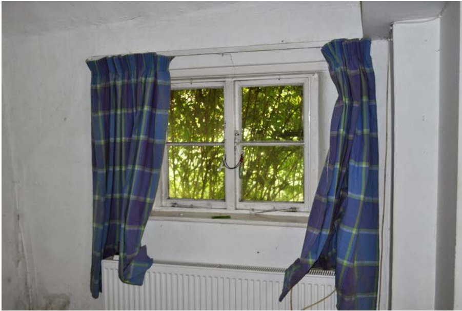
Plate 37: Window W4 in room 6.
