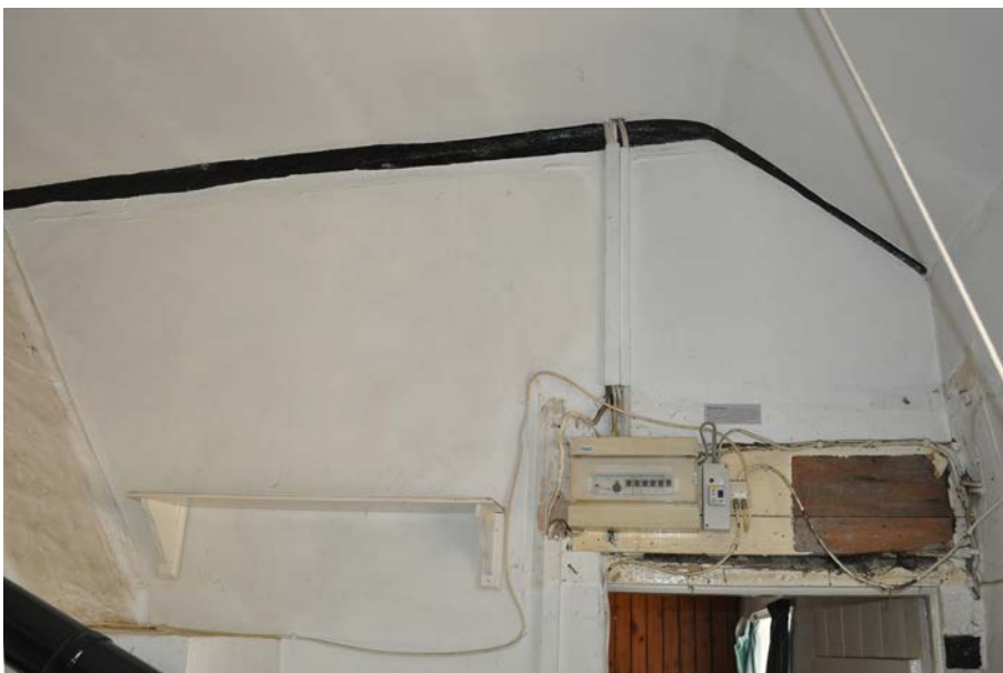
Plate 30: West side of Room 3 showing exposed timbers.
