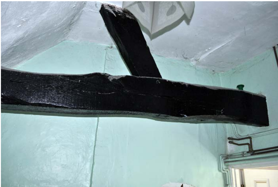
Plate 32: Exposed part of Truss 3 in Room 4.
