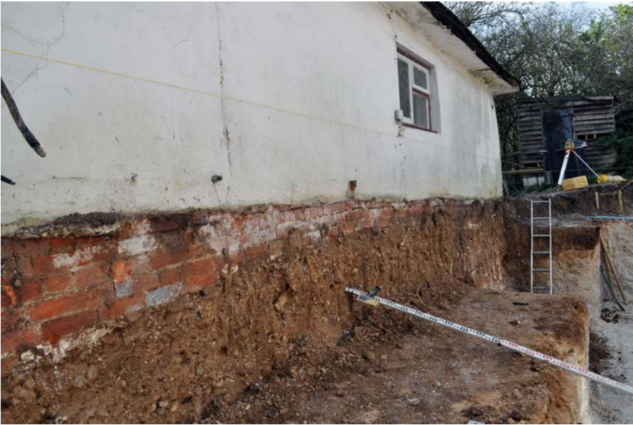
Plate 13: Detail of brick footings looking west.
