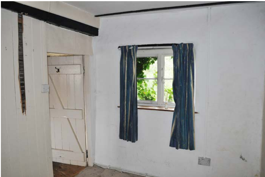
Plate 23: South side of Room 2 with window W1 and door D2.
