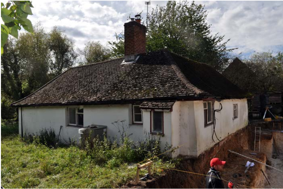
Plate 4: North and east external elevations of cottage, viewed from ENE.
