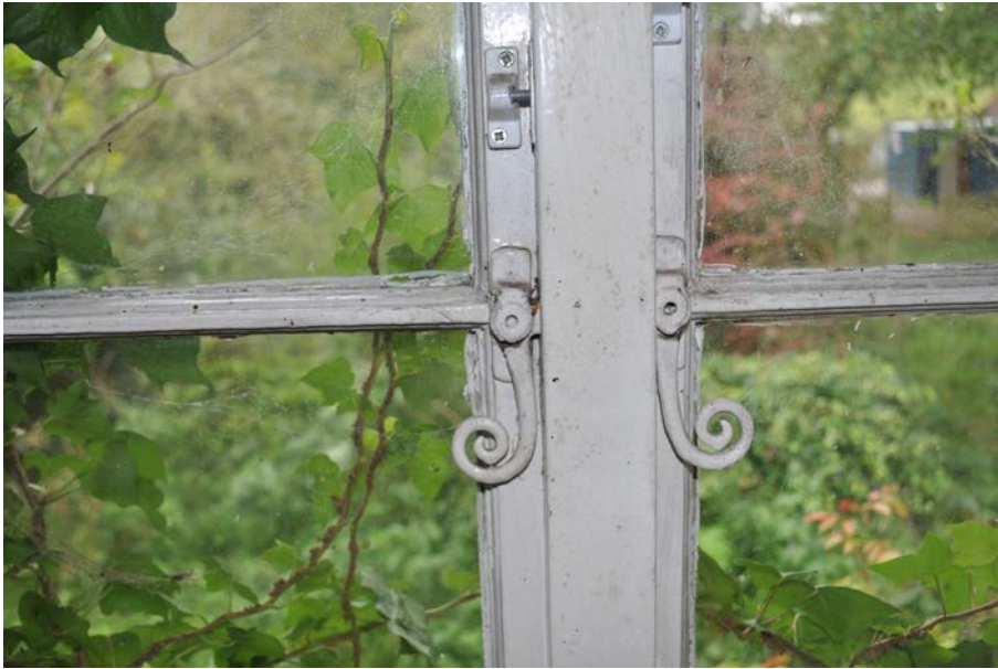
Plate 25: Detail of window catches on window W1.
