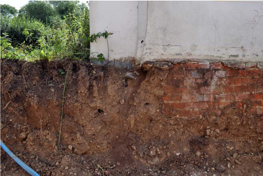
Plate 14: Detail of east end of footings of north elevation.
