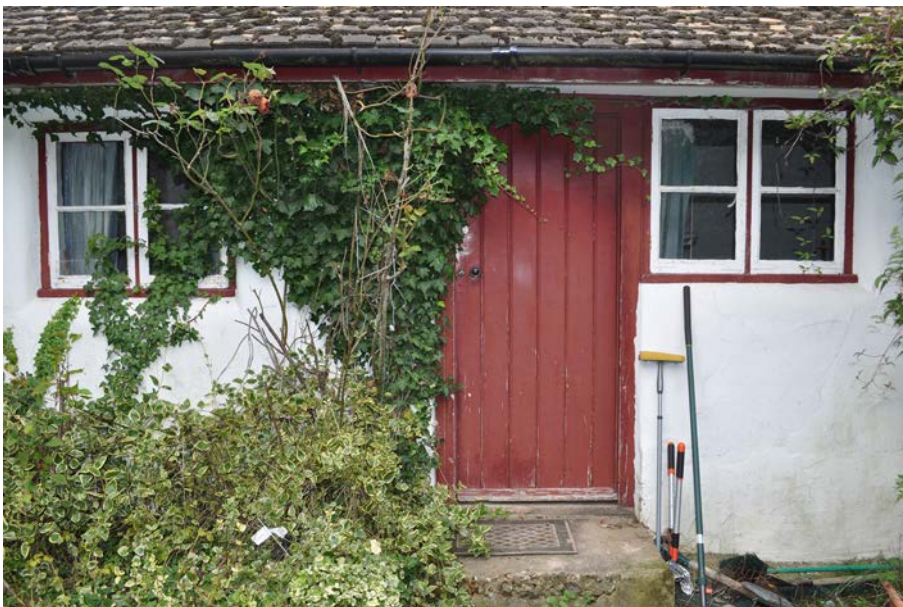
Plate 5: Door D1 and windows W1 and W2 in south external elevation.
