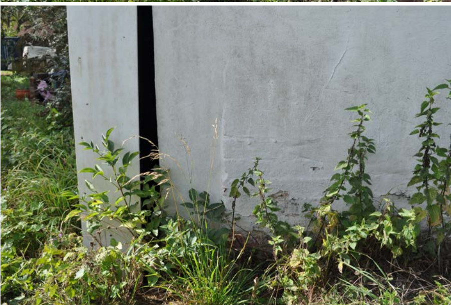
Plate 9: Detail of south end of east elevation showing painted brick-work.
