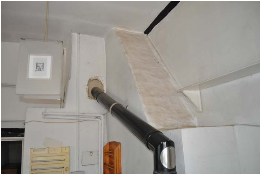
Plate 29: Detail of L-shaped flue in SW corner of Room 3.
