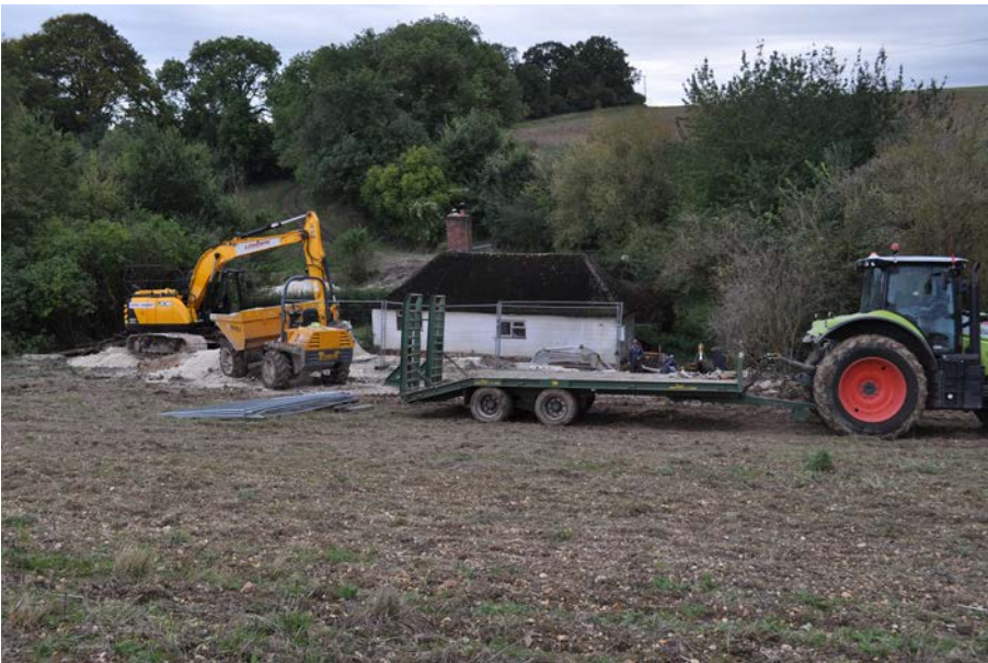
Plate 2: View of cottage set in dip in landscape, looking south.
