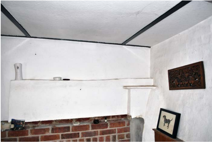
Plate 19: Detailed view of probable blocked fireplaces in east wall of Room 1.
