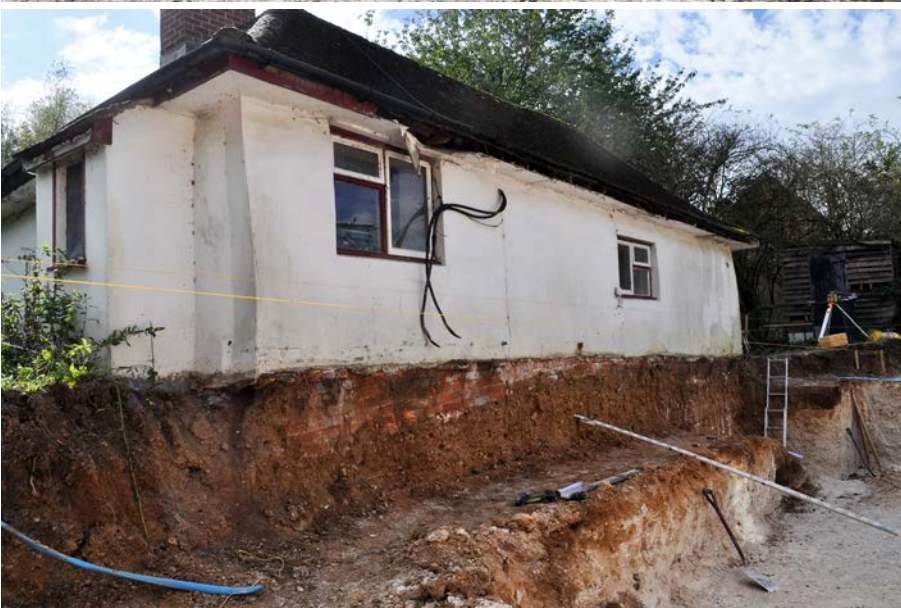
Plate 12: North external elevation showing brick footings below cottage revealed in groundworks for new extension. Viewed from ENE.
