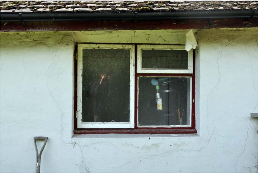
Plate 10: Window W5 in east elevation.
