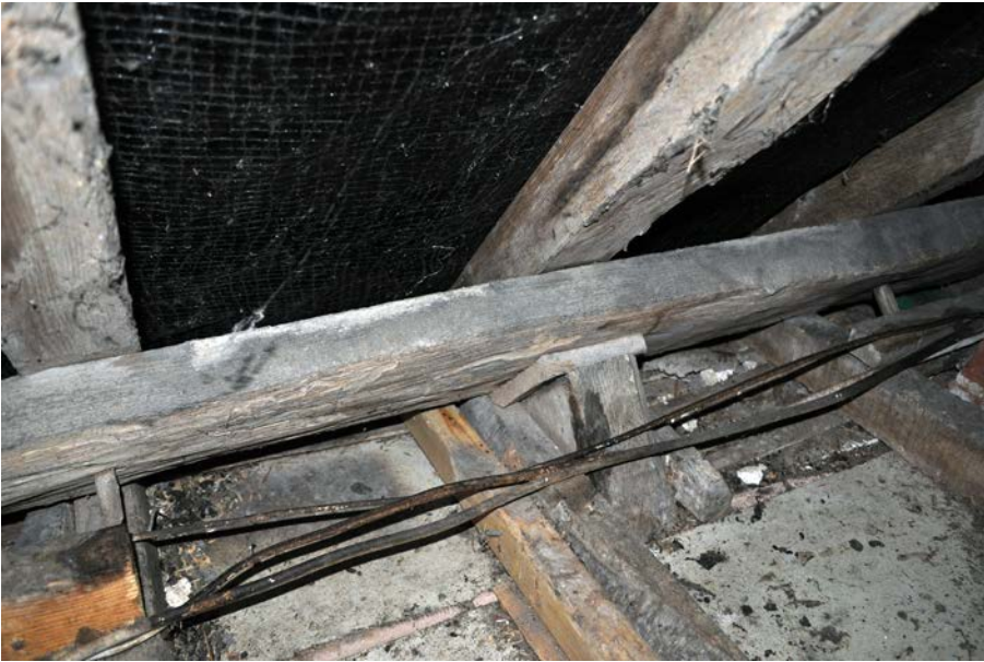
Plate 40: Detail of west end of Truss 3 visible in roof space.
