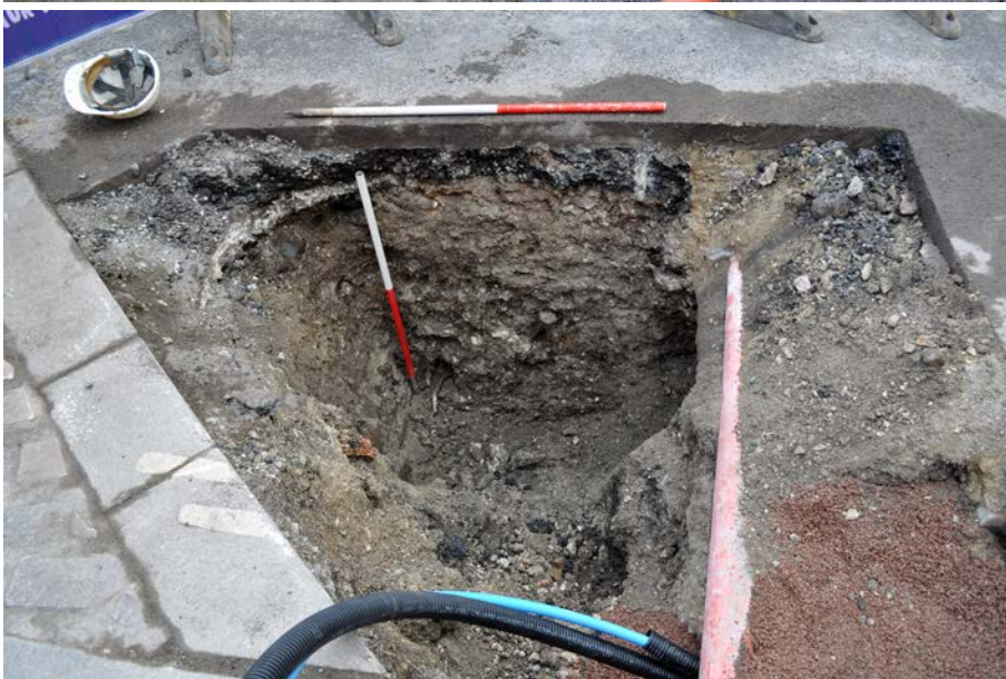
Plate 6: Trench in road showing soil layer 106. 1m scale.
