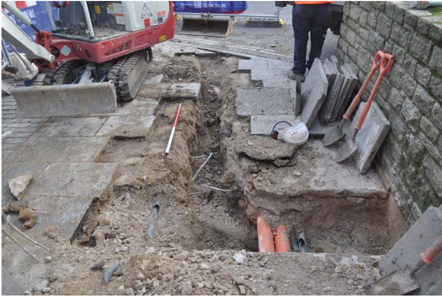
Plate 4: Trench in pavement after excavation, looking east. 1m scale.
