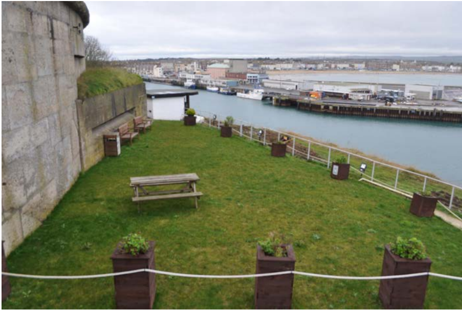
Plate 1: View westwards from the upper slope of the north terrace, with the excavated drain trench just beyond the metal fence.
