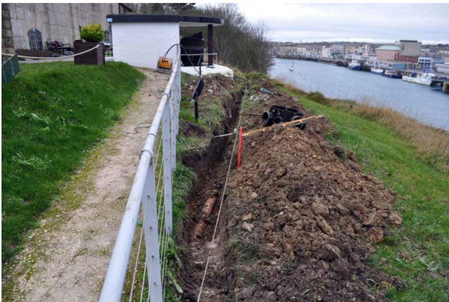
Plate 2: View of the emptied existing drain trench, looking east. 1m scale.
