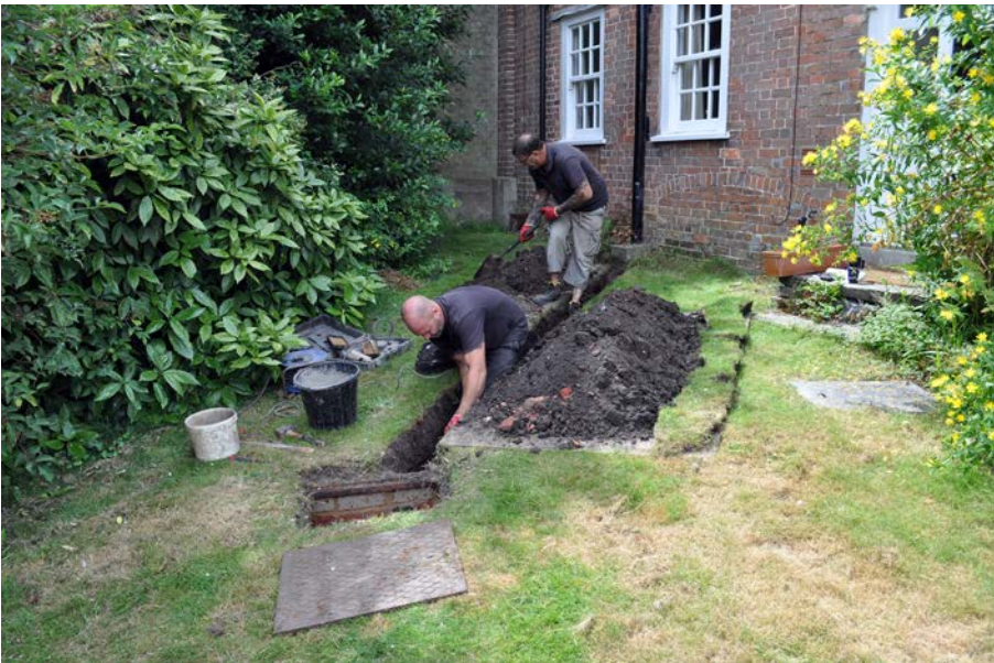
Plate 5: Trench 3 during excavation, looking south west.
