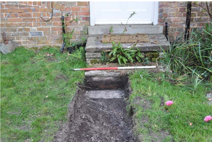
Plate 14: Step 602 in Trench 6, looking west. 1m scale.
