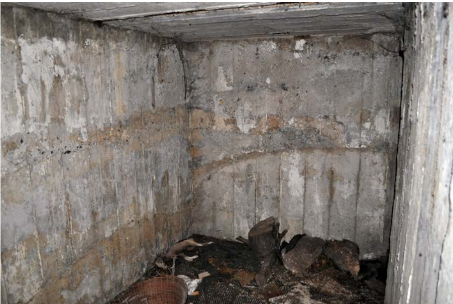
Plate 17: Interior of air raid shelter, looking south.
