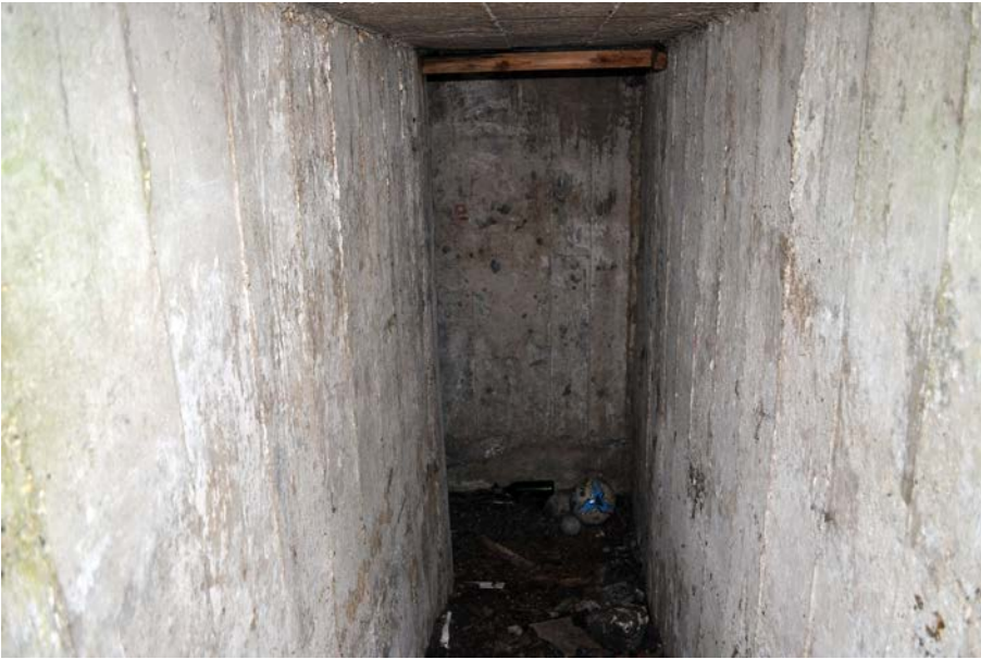
Plate 16: View along corridor from north entrance of air raid shelter.
