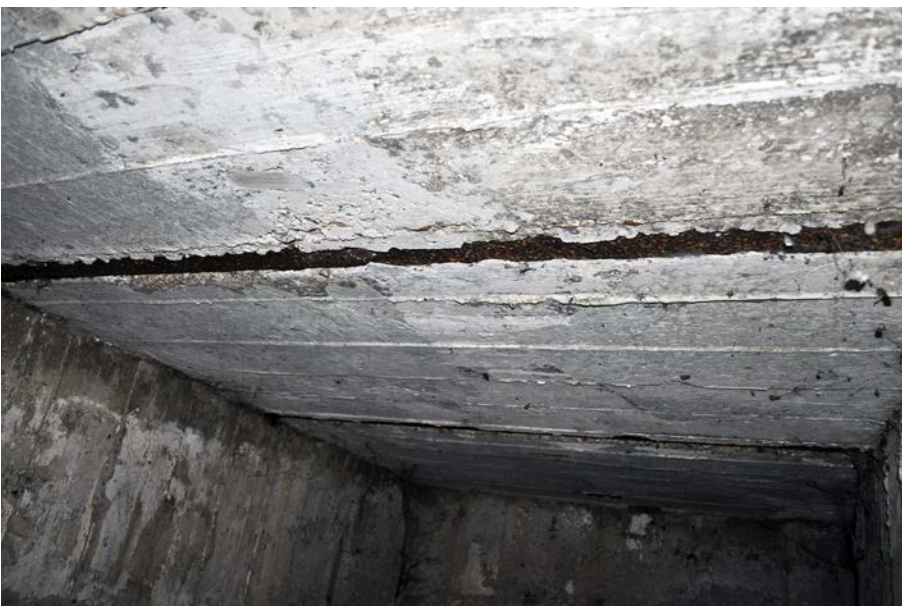
Plate 18: View of roof in interior of air raid shelter, looking south.
