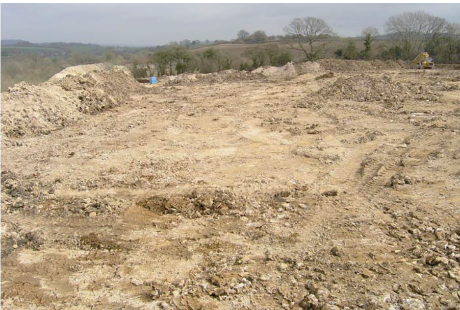
Plate 3: View of the north end of the site from the west.
