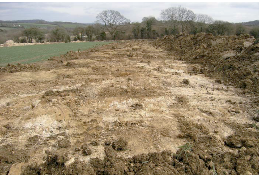
Plate 2: View of the south end of the site from the west.
