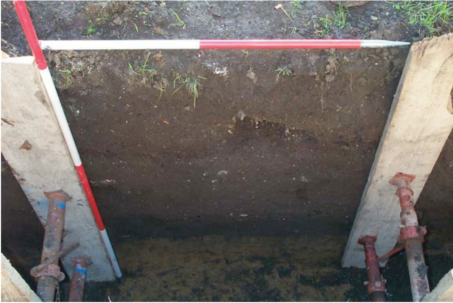
Plate 9: Trench 5 – West facing section detail from east arm of footings trench.
