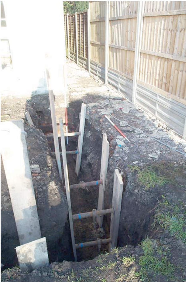
Plate 5: Trench 5 - Northern arm of footings trench.
