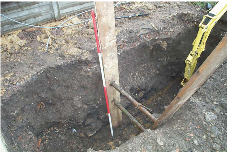
Plate 10: Trench 5 – West end of north arm of footings trench.
