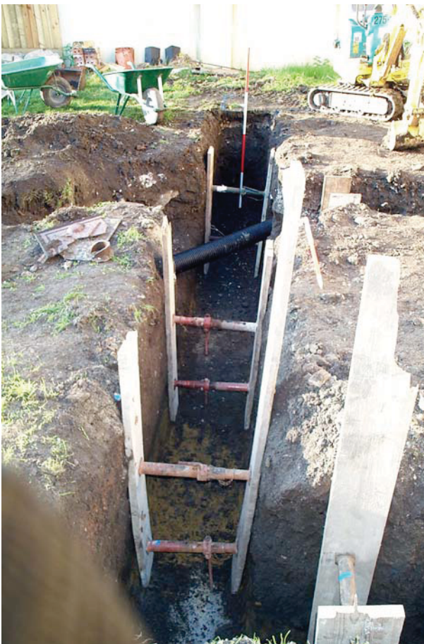
Plate 8: Trench 5 – East arm of footings trench.
