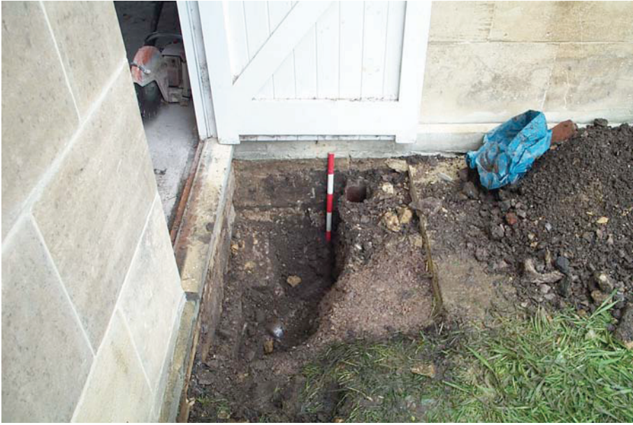
Plate 4: Test Pit 4 – east-facing section.
