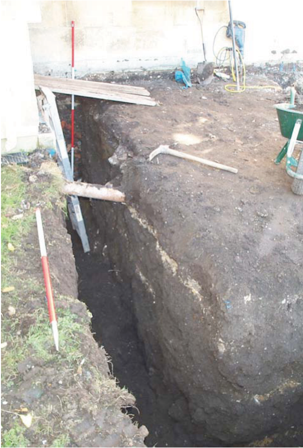
Plate 7: Trench 5 – South arm of footings trench.
