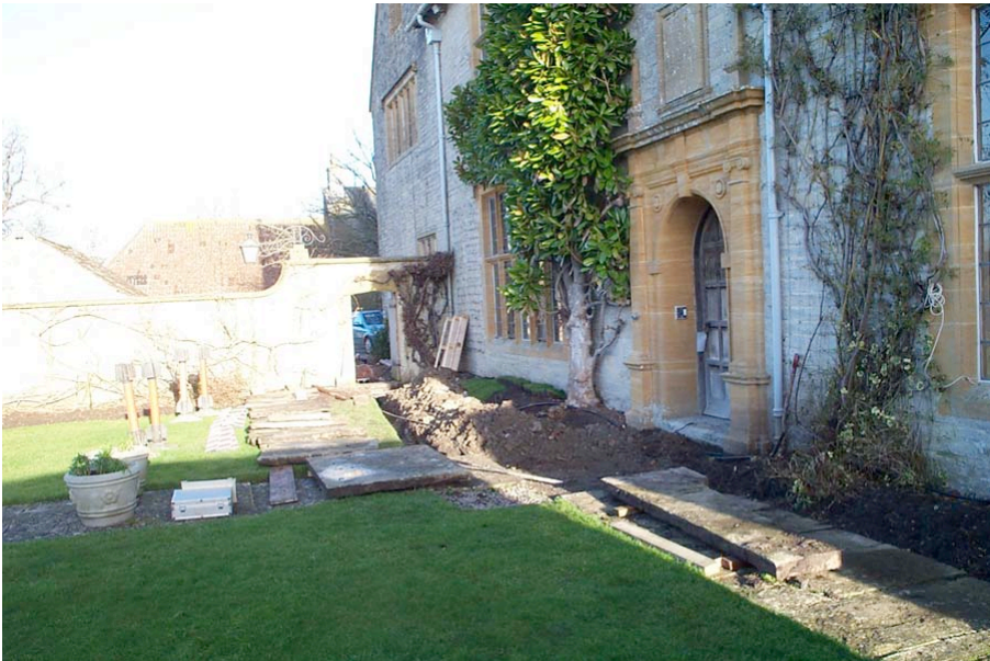
Plate 2: General view of Trench 2 along West Wing of Lytes Cary House, looking North.
