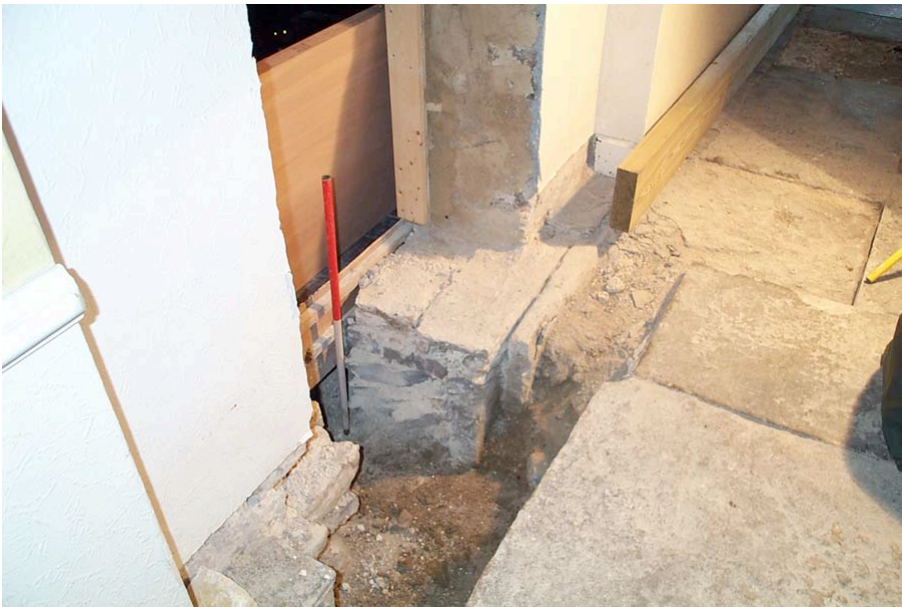
Plate 7: View of trench cut through wall footings 119.
