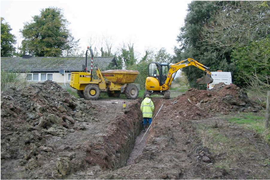
Plate 1: General view during excavation of foul drain trench (Trench 1), looking North.
