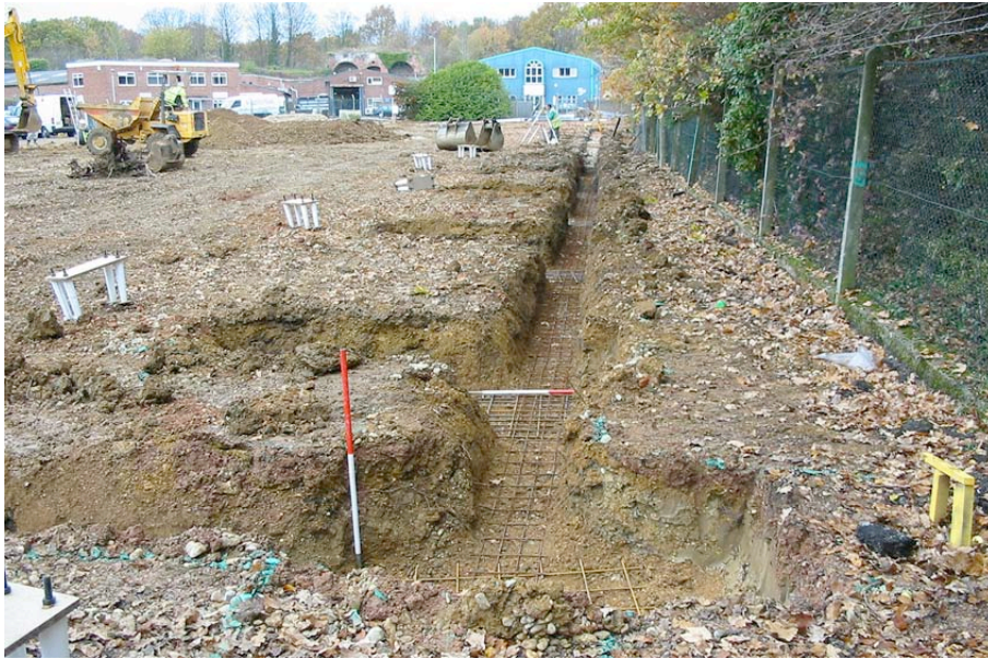
Plate 7: East side of Trench 3, looking north.
