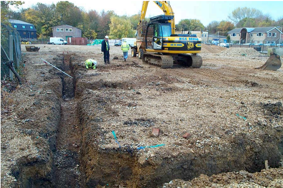
Plate 4: Eastern side of Trench 2, looking south.
