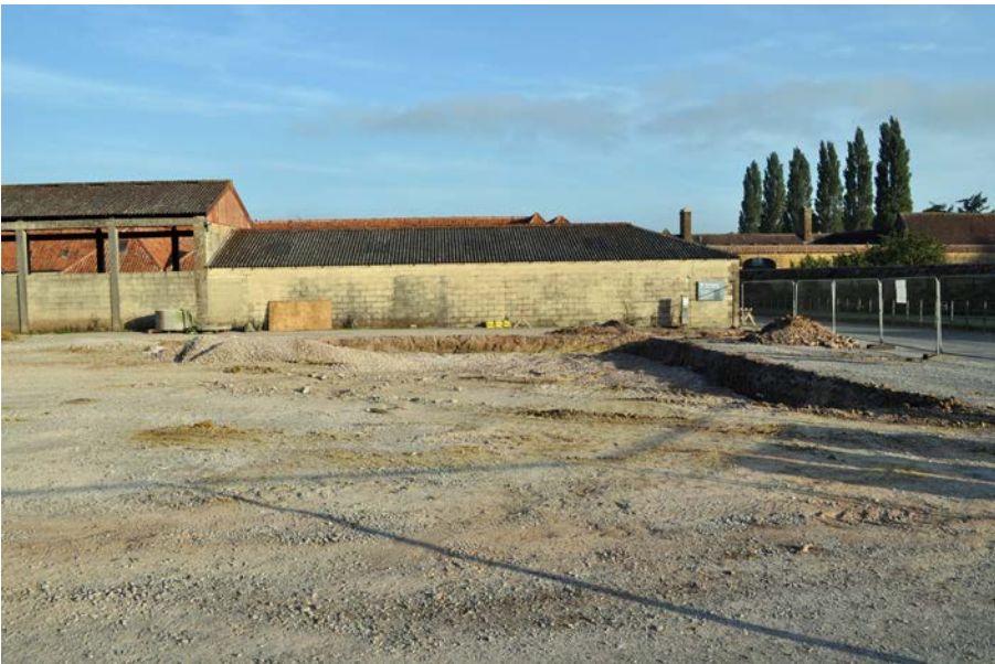
Plate 8: Beagles Car Park, showing drainage trench, looking north.
