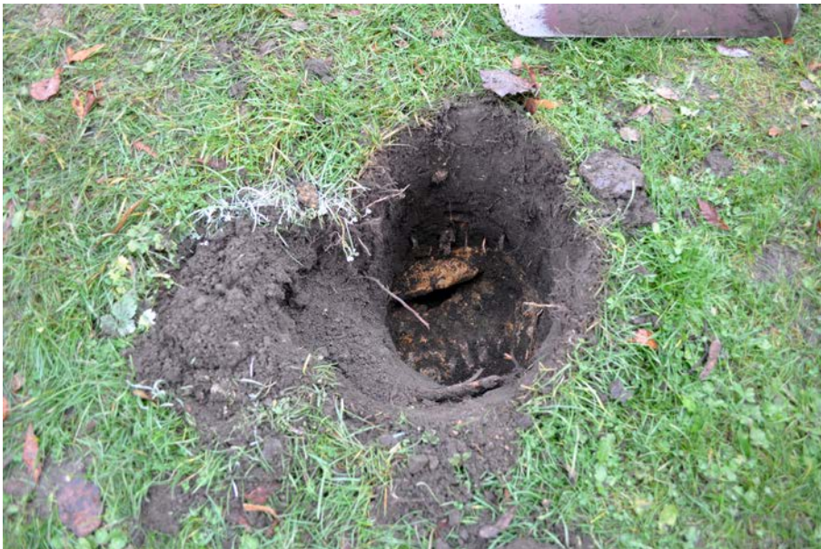
Plate 5: Trench 2 after excavation showing stone drain 104 in base of hole, looking east.
