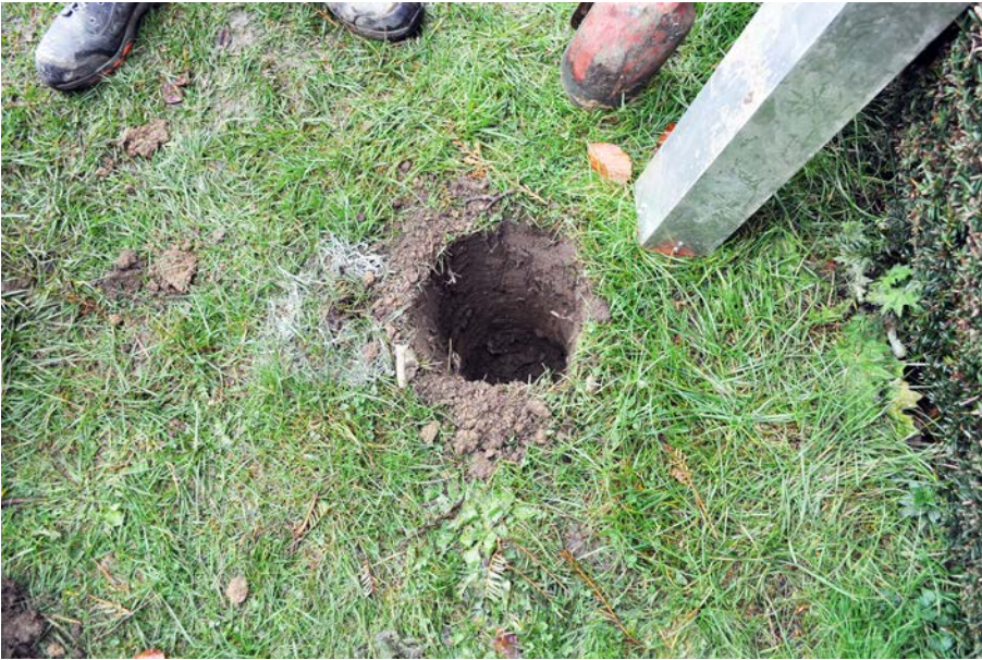
Plate 7: Trench 3 after excavation, looking south.
