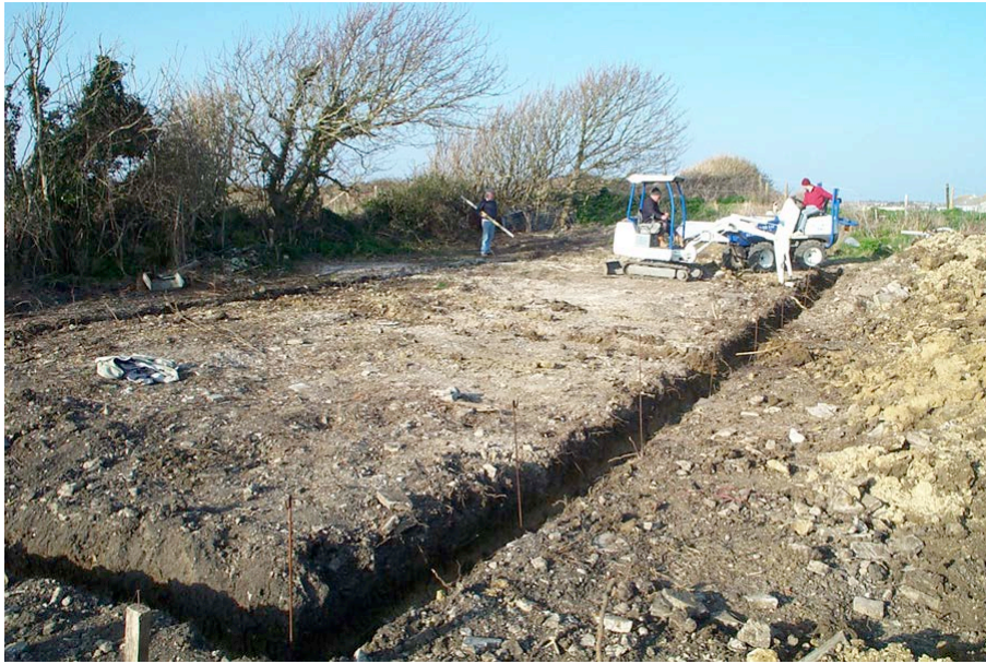
Plate 1: View of site during excavation of footings trenches, viewed from south.
