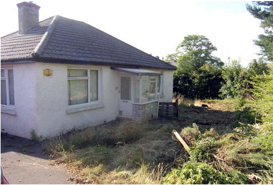
Plate 1: 69 Mount Pleasant Avenue South prior to evaluation trenching. View from north west.
