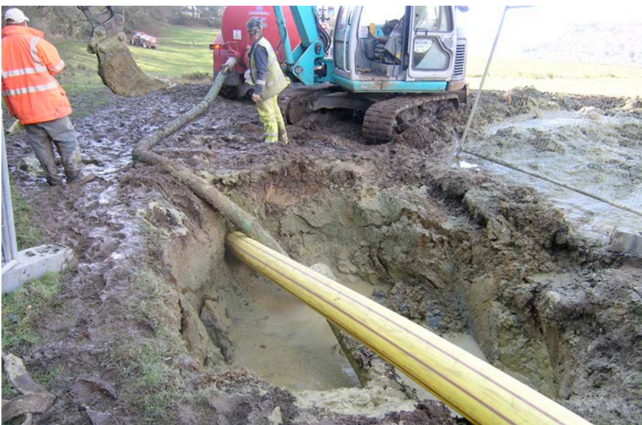
Plate 12: Trench 52 during insertion of gas pipe.
