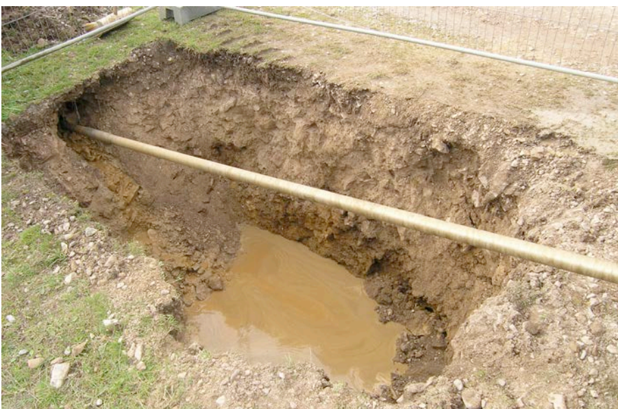
Plate 6: Trench 21 viewed from SW showing topsoil over natural deposits.
