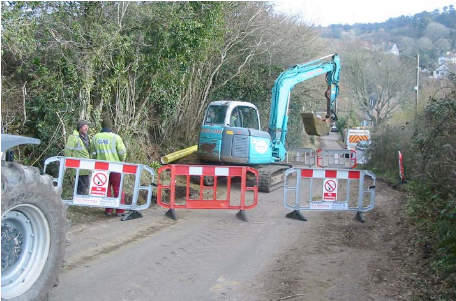
Plate 1: View NE down Ship Knap during excavation of Trench 5.
