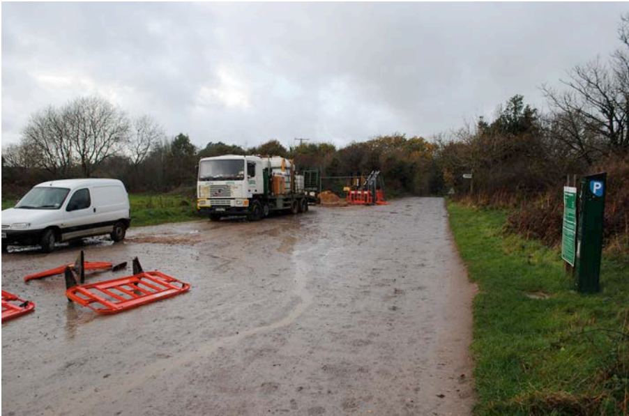
Plate 7: Drilling operations in Stonebarrow Hill car park looking east towards Trench 32.
