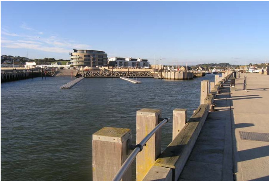
Plate 10: View of West Bay outer harbour from the east pier.
