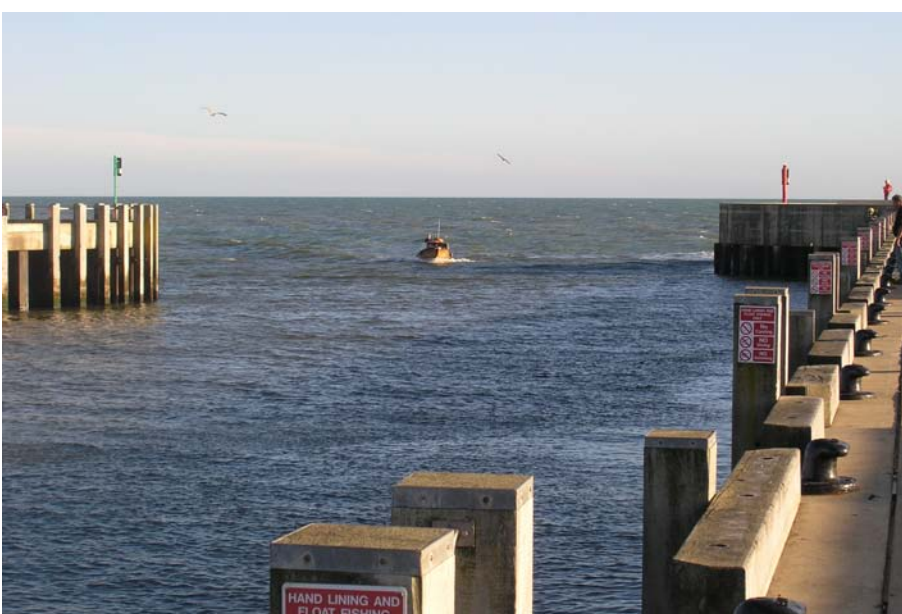
Plate 11: View of West Bay harbour entrance from the west pier.
